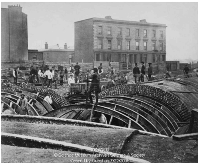
Figure 3.29 Site construction of the Victoria Street, Blackfriars, 1869
