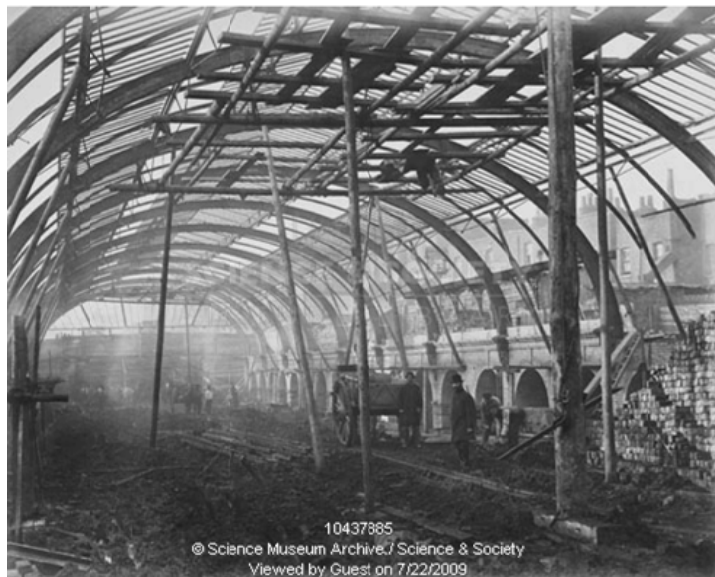
Figure 3.30 Construction of Bayswater Underground Station, 1867
