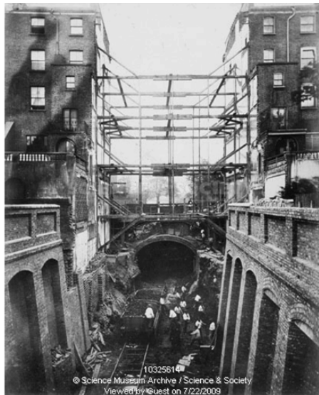
Figure 3.27 Construction of the Metropolitan District Railway, Bayswater, 1867
