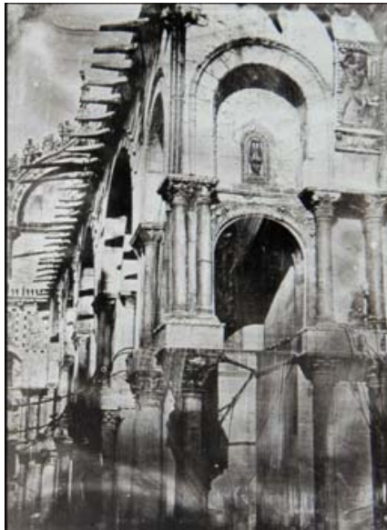
Figure 2.6 North-West Porch of Basilica of St. Mark by Ruskin, 1850-1851
