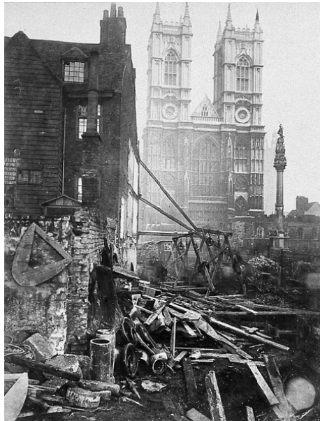
Figure 3.26 Construction of the Metropolitan District Railway, Westminster, 1869
