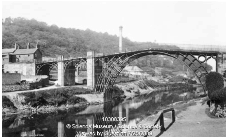
Figure 3.34 The cast iron bridge over the River Sever, Coalbrookdale by unknown photographer, late 19th century
