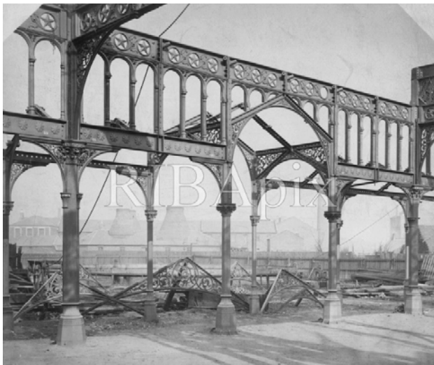
Figure 3.39 Central Market, Santiago: view of the prefabricated structure being assembled in Britain before shipment to Chile, 1860s
