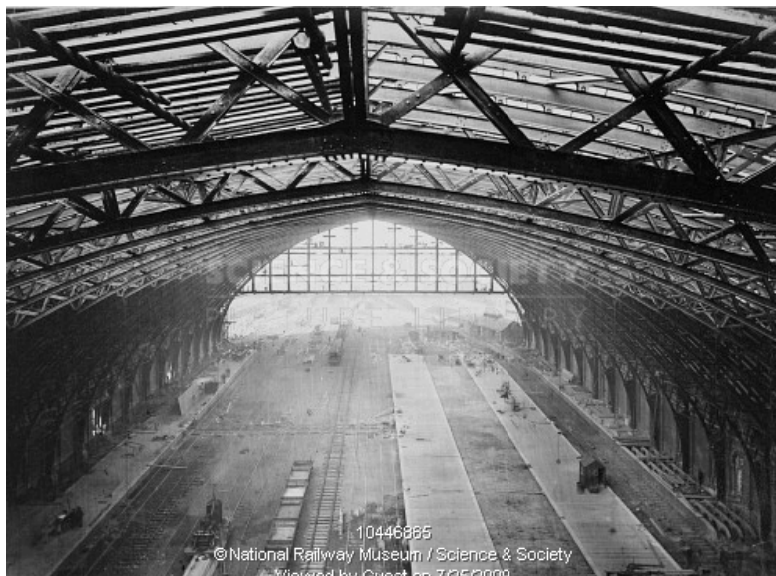
Figure 3.41 Arched Train Shed of St Pancras Station, 1868
