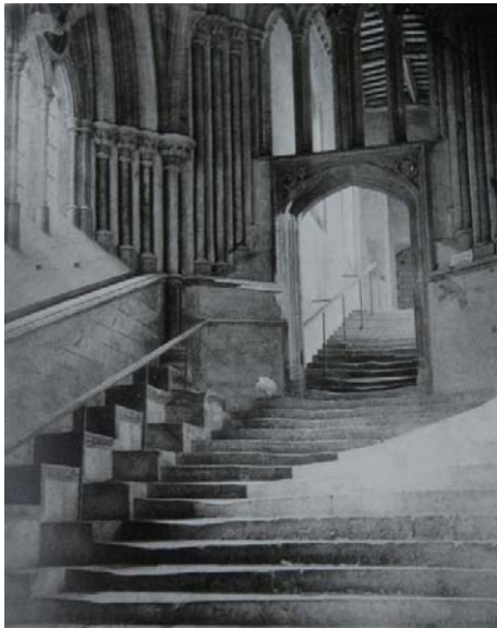
Figure 3.11 Stairs of Wells Cathedral by Cundall, 1862
