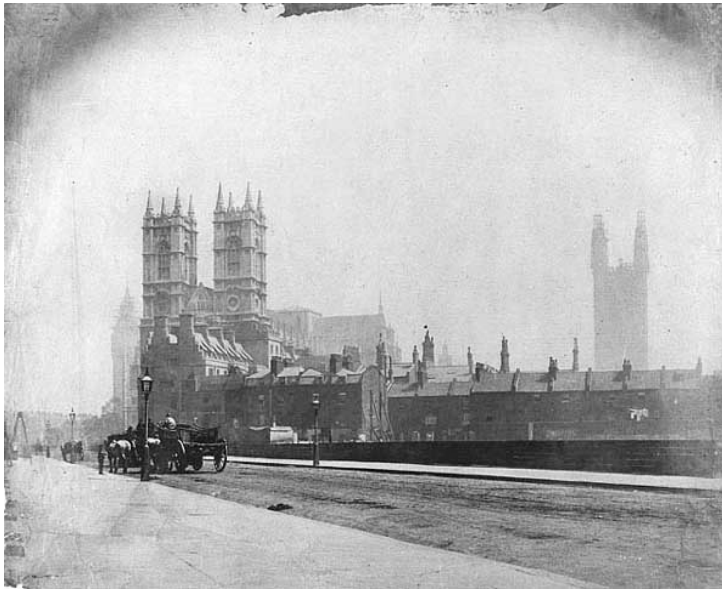
Figure 3.20 Westminster Abbey looking towards the Houses of Parliament under construction, by Roger Fenton, 1857
