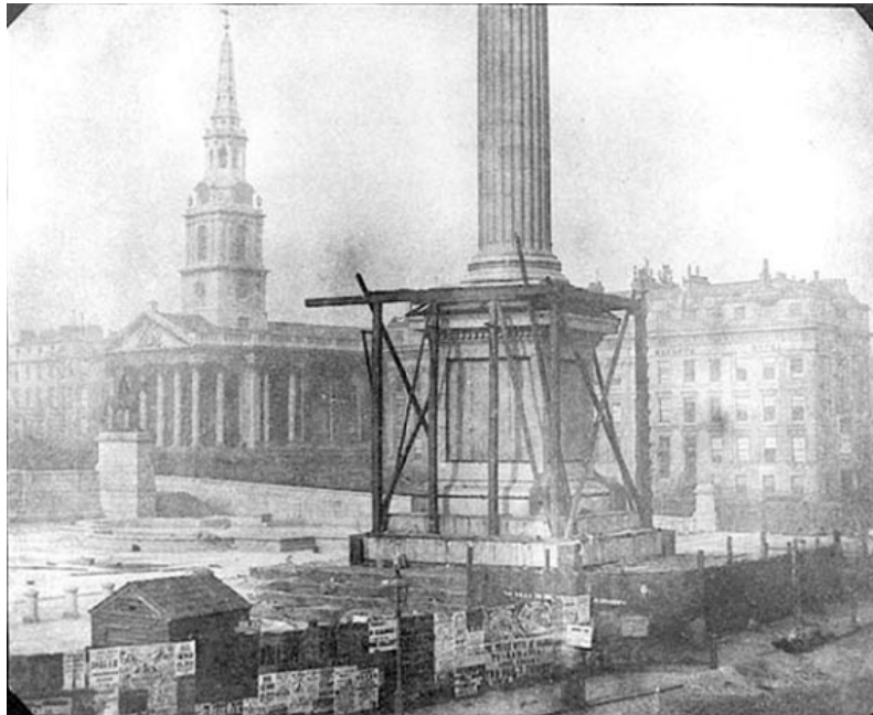
Figure 3.18 Trafalgar Square, Nelson Column by Talbot, 1843
