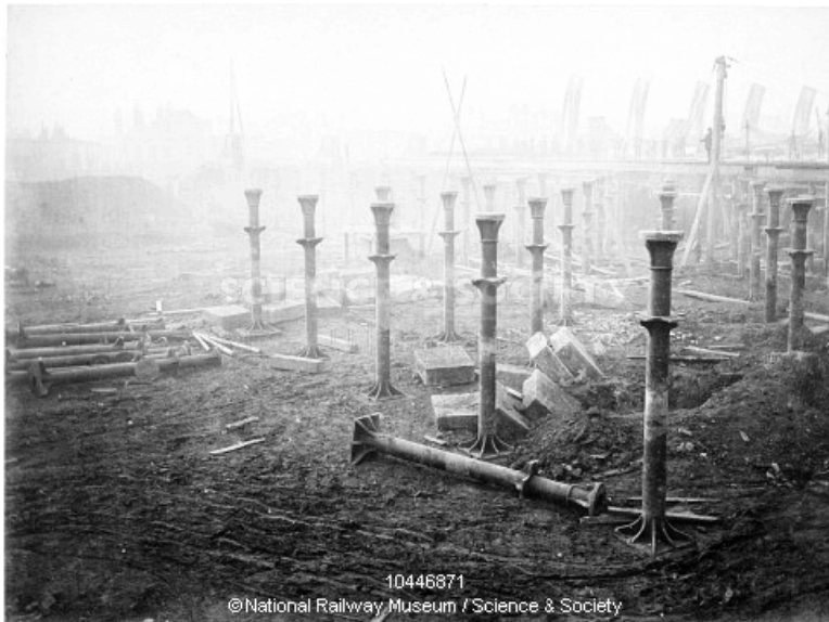
Figure 3.40 General view of the construction of St Pancras station, 1867
