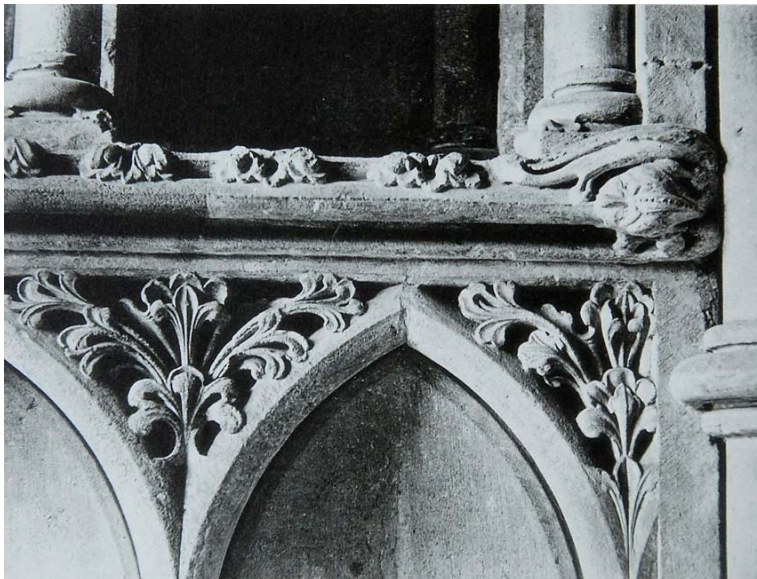
Figure 3.10 The part of nave triforium by Joseph Cundall, 1862
