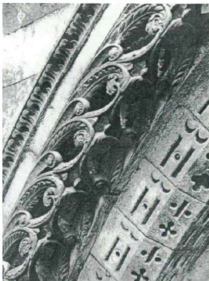
Figure 2.7 An architectural detail, from St. George's Collection, 1870s
