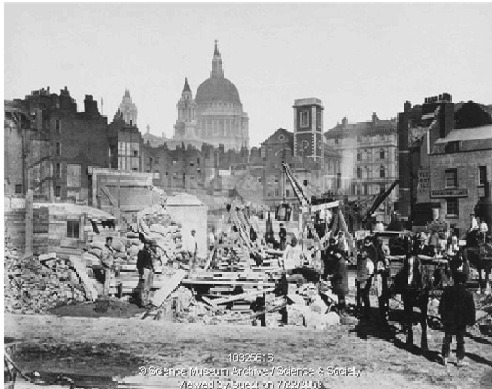
Figure 3.28 Site clearances at Queen Metropolitan District Railway, 1867
