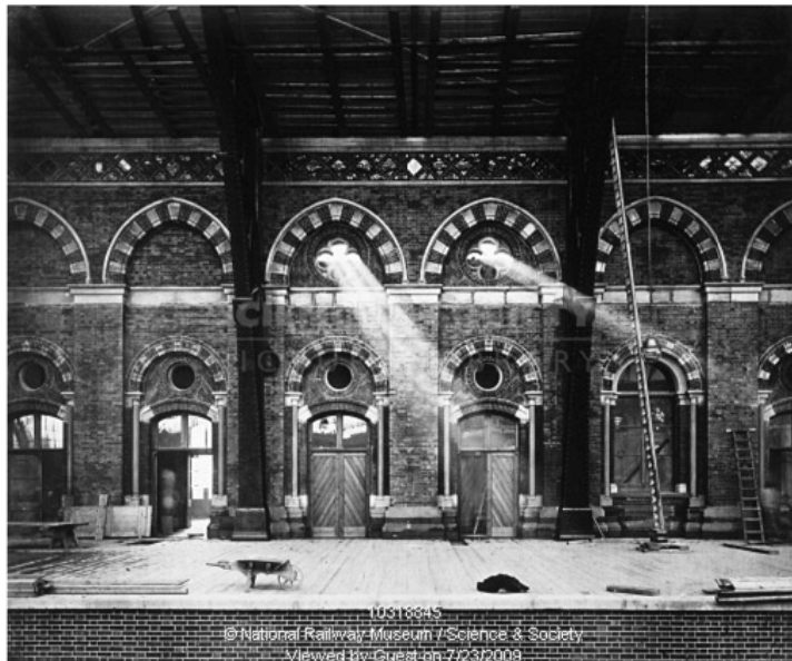
Figure 3.16 St Pancras Station
