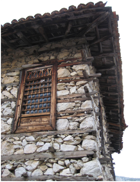
Fig.1.6. (left) The architectural dimension of the cultural tradition is illustrated by the characteristic construction technique of the Akseki-İbradı Basin. This thesis will call this technique as “timber reinforced rubble stone masonry with projecting tie beams”. The photograph indicates the façade of a traditional dwelling in Ormana (photograph by K.R. Kavas)
