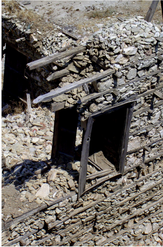
Fig.1.12. A collapsed traditional structure in the Orta District of Ürnlü indicates the sectional configuration of the characteristic timber reinforced rubble stone masonry. (photograph by K.R. Kavas)
