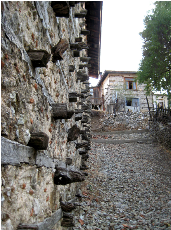
Fig.2.14. The projecting tie beams (peştivan) constitute the characteristic spatial qualities of environment. (Ürünlü) (photograph by Kemal Reha Kavas)
