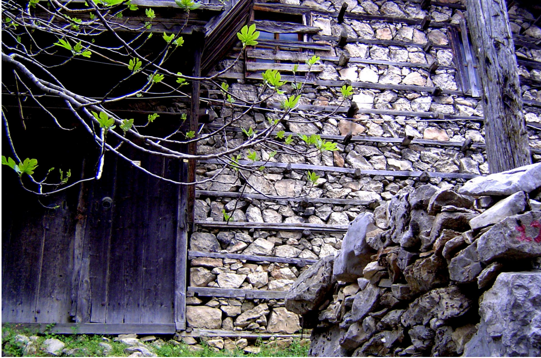
Fig.2.13. The characteristic construction technique of the Akseki-İbradı Basin, Timber-reinforced rubble stone masonry, is the sustainer of the environmental coherence in Ürünlü. (photograph by Kemal Reha Kavas)
