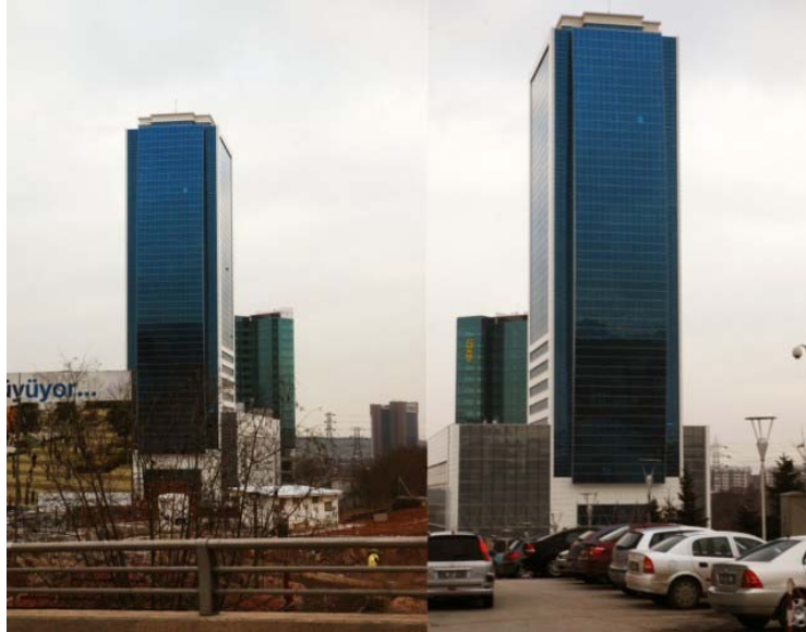
Figure 14. Bayraktar Tower (photographed by the author on 06.03.2009)
