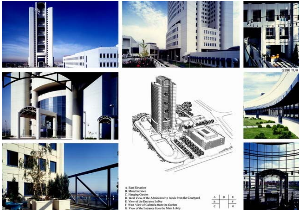
Figure 44. Halkbank Headquarters - Views
