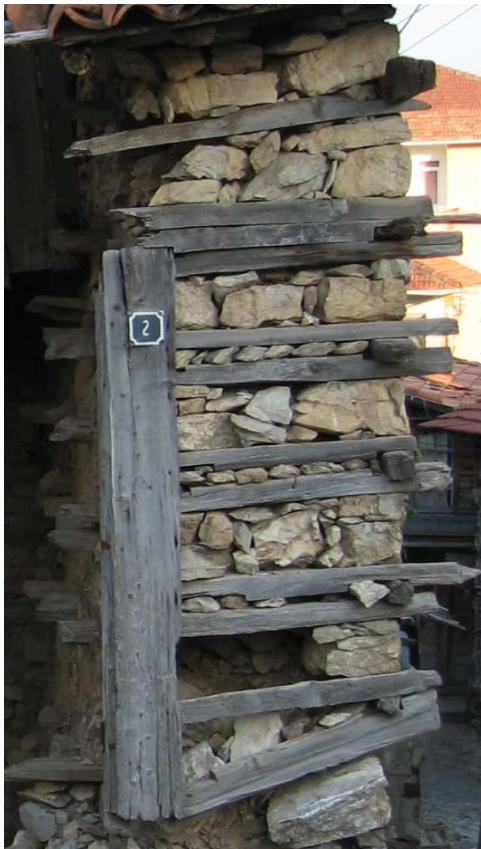
Figure 4. 14 Detail from the wall connection. Çelik 2008.
