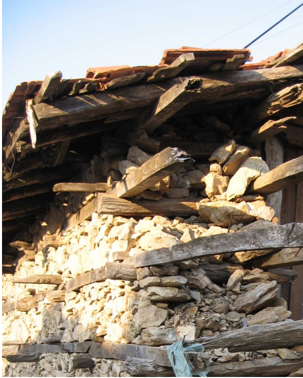
Figure 4. 42 Detail from the roof-wall connection. Çelik 2008.
