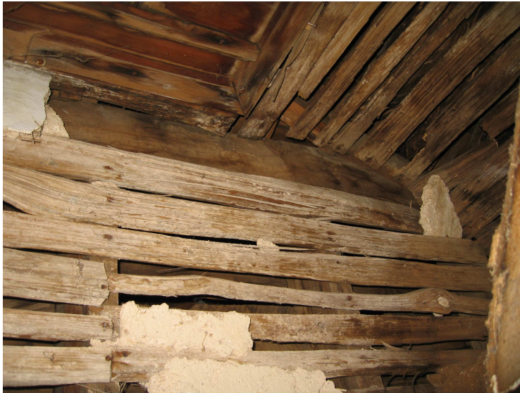
Figure 147 View from wood lath wall of the Eyüpoğlu House. Çelik, 2008.
