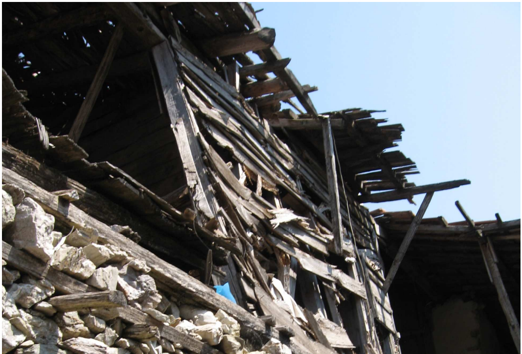
Figure 4. 21 Detail from timber wall type 4. Çelik 2008.
