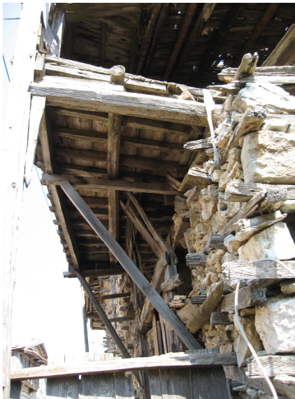
Figure 4. 32 Detail from the projection type 1 Çelik 2008.
