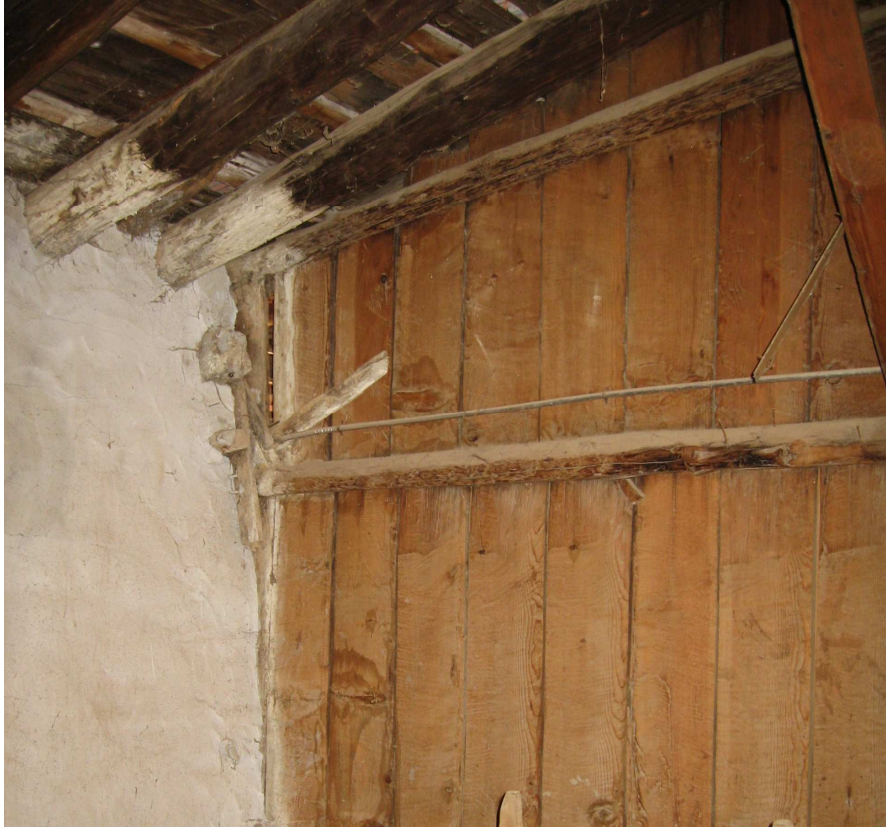
Figure 1 Detail from timber wall type 2. Çelik 2008.
