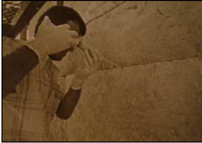
Figure 3.6. Leaking of the grout between the fragments of the Northwest Heroon, Sagalassos (Source: Wealkens, M. Ercan S., Torun E., 2006)
