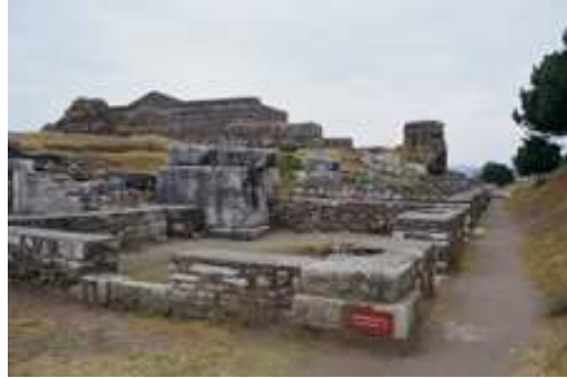
Figure 3.23. Capping of the walls of the Byzantine shops, Sardis, 2003.
