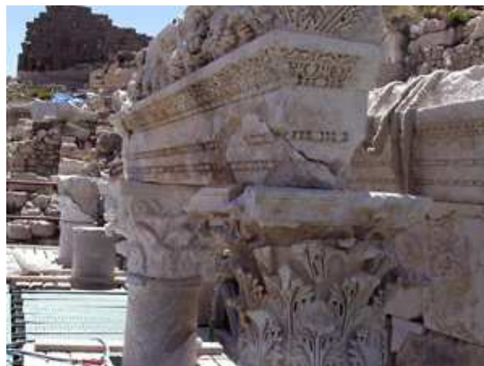
Figure 3.5. New Corinthian capital carved from original material from the second aedicule, Sagalassos (Source: Accessed by http://www.archaeology.org/interactive/sagalassos/field06/antnymph1.html on March 18, 2009)
