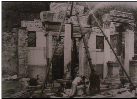
Figure 4.18. Use of casts in white instead of the damaged original pieces, 1957 (Source: Wiplinger, G. & Wlach, G., 1995, p.72).
