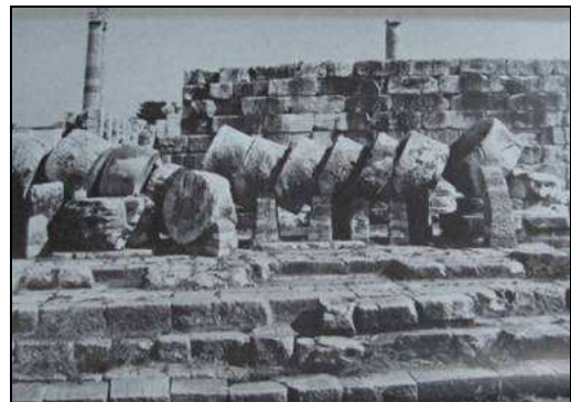
Figure 2.3. The missing column shafts designed as short elements at the Trajan Fountain, Ephesus.
