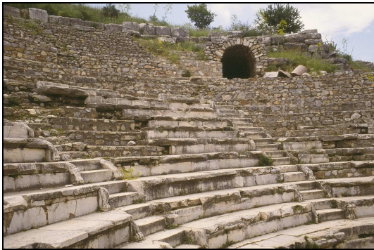
Figure 2.9. The seating blocks of the Bouleterion completed with rubble stones, Ephesus.
