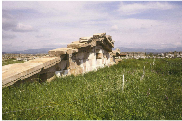
Figure 3.3 Use of concrete (with black cement) in the terrace façade of the Domitian Temple, Ephesus (Sources: Scherrer, P., 2000, p.93).
