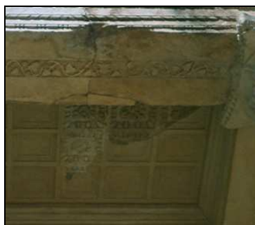
Figure 2.26. The new and authentic parts of the coffins of the Tetrapylon, Aphrodisias.
