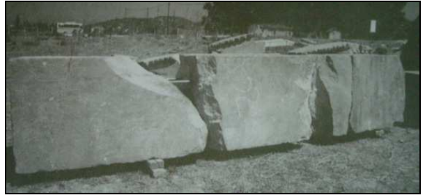
Figure 3.6. Leaking of the grout between the fragments of the Northwest Heroon, Sagalassos (Source: Wealkens, M. Ercan S., Torun E., 2006)
