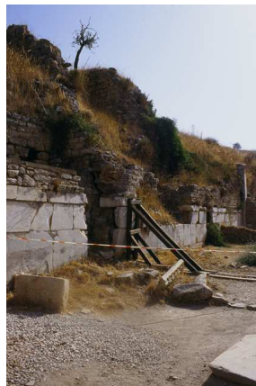
Figure 3.28. Supporting the leaning wall of the basilica stoa, Ephesos, 2003
