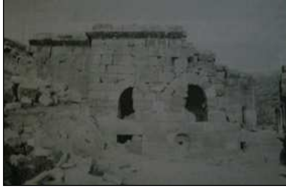
Figure 3.34. Consolidation of the leaning wall at the north of the Theater, Hierapolis (Source: Bernardi, D.F., 1995, p.348)
