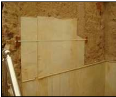
Figure 4.8. The marble panel fixed with band, 2008.
