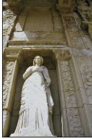
Figure 3.8. The missing parts of the ornamented blocks at the east façade of the Celsus Library, Ephesus.
