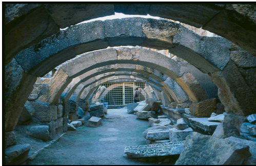
Figure 2.5. The arches of the proskene completed with concrete (with black cement) at the Theater, Hierapolis
