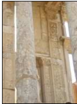
Figure 4.28. The colors of the missing parts similar with original elements
