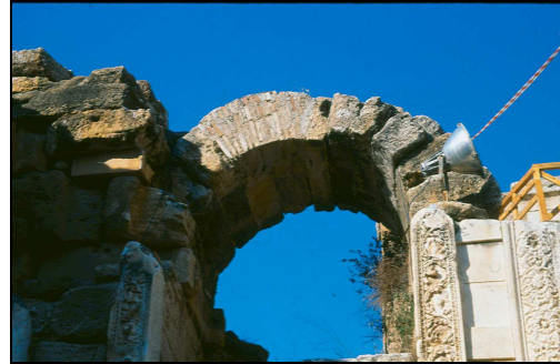
Figure 2.5. The arches of the proskene completed with concrete (with black cement) at the Theater, Hierapolis
