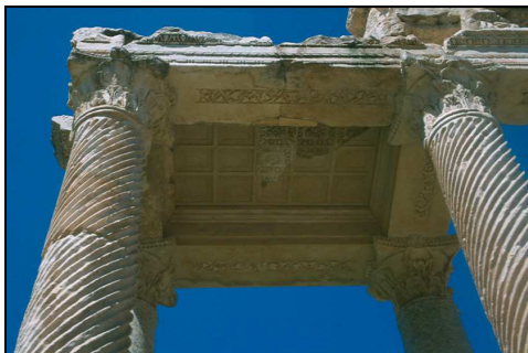
Figure 2.11. Consistent intervention in the coffins of the Tetrapylon, Aphrodisias.
