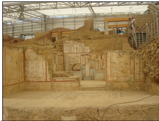
Figure 4.15. Consistent treatments on the top of the walls
