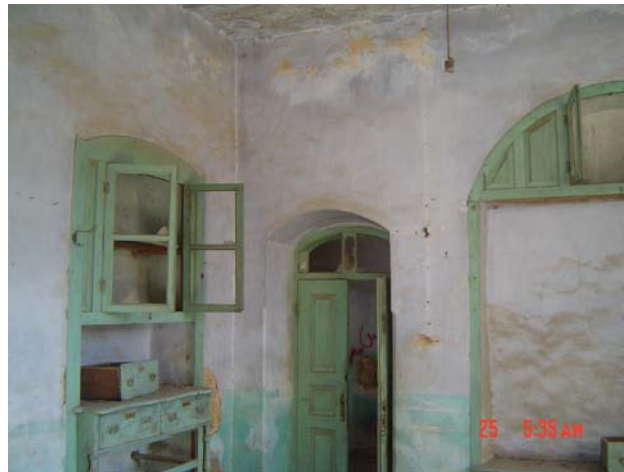
Figure 11.6: space 0.6, south-east corner
