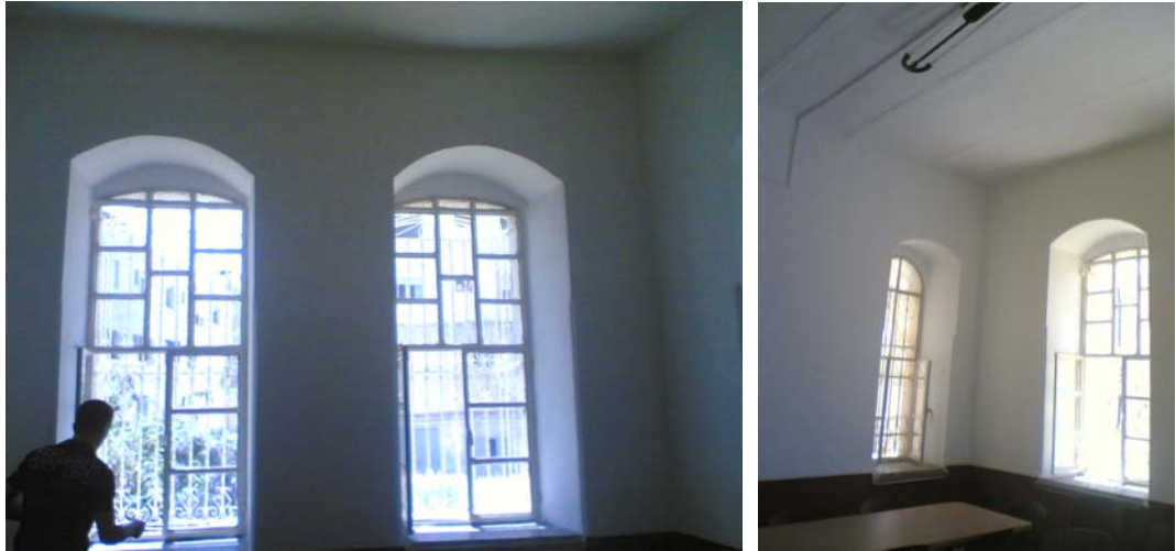
Figure 9.9: space 1.7, looking west and south-west directions
