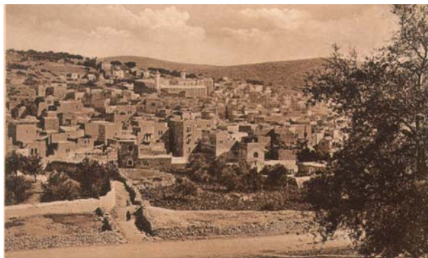
Figure 50: view of the traditional town from the south-west direction Source: taken in 1890, HRC archive.
