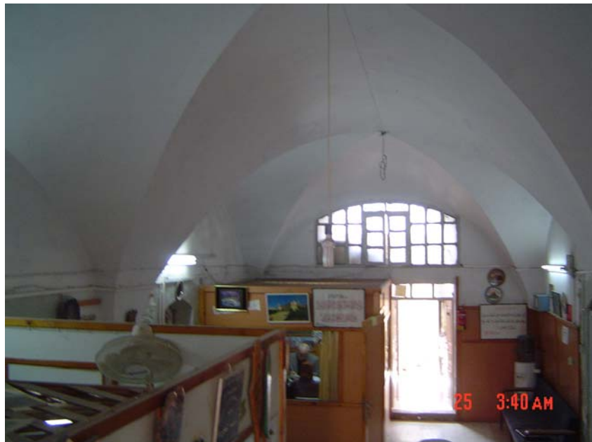
Figure 4.6: space 0.1, south wall
