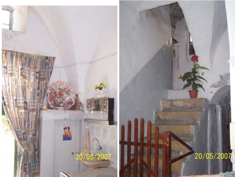
Figure 17.3: space 1.1, looking south-west, and then looking stairs leading to north exit
