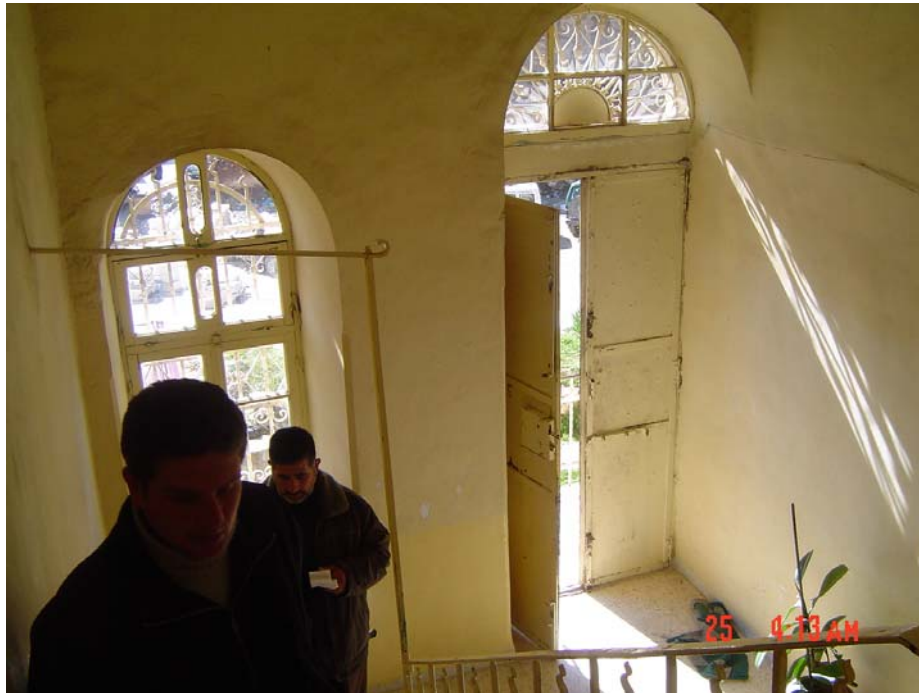
Figure 2.6: space 1.5 staircase space to first floor
