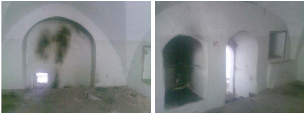
Figure 14.6: space 0.5, on the left looking south-east corner, then north wall
