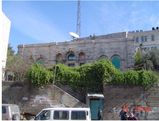
Figure 72: main (west) elevation, Yosef Abu-Snaynih house, Jerusalem Road
