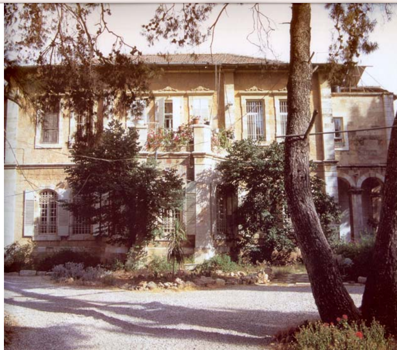
Figure 104: Saied Hosayni - Jerusalem constructed in 1902. Ground floor plan and north (main) elevation photograph
