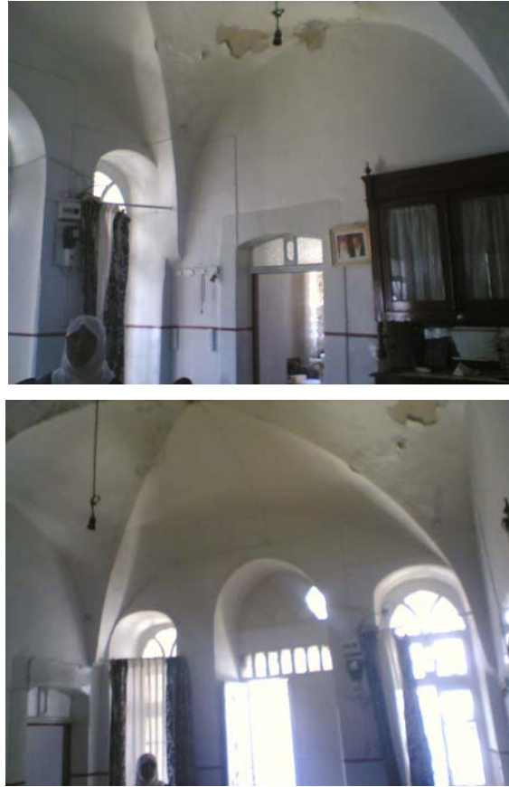
Figure 7.6: space 1.1, looking north-west corner then looking west wall
