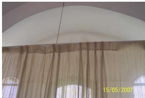
Figure 18.8: space (0.1), looking east wall
