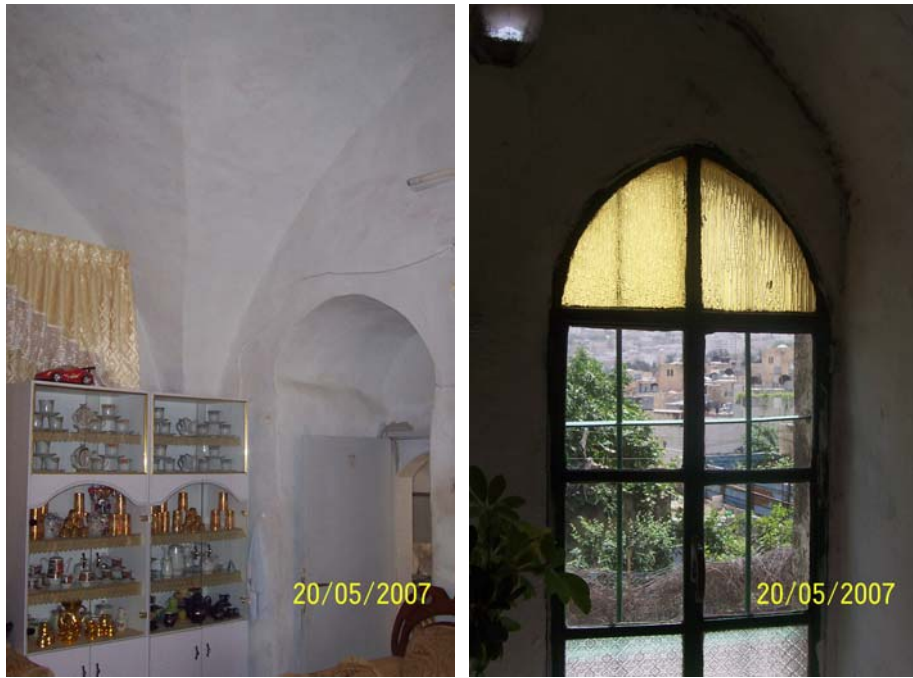
Figure 17.5: space 1.3, on the left looking south west corner, on the right looking east wall window
