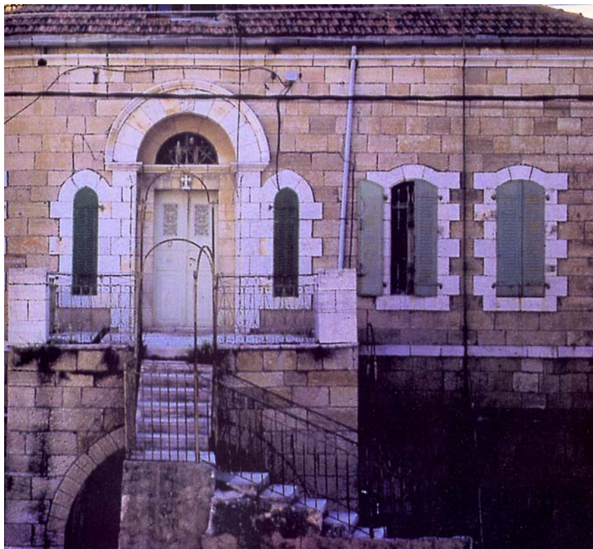
Figure 91: Ibrahim Salem Issa house-Ramallah constructed in 1911. Plan, elevation, and then main elevation photograph
