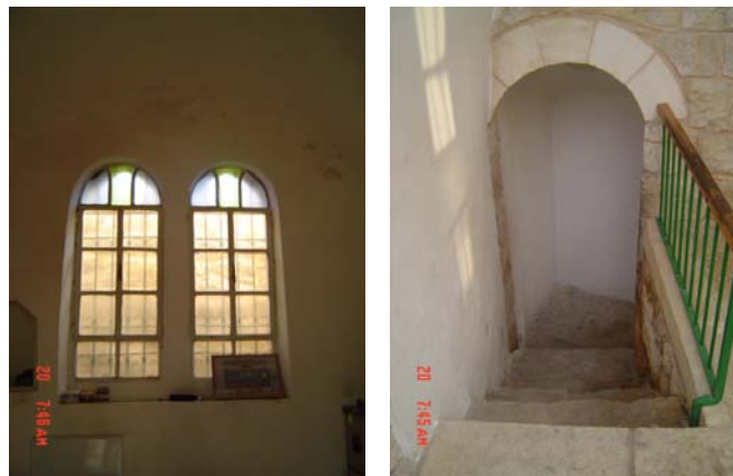
Figure 19.5: space 1.7 south wall window, then space 2.2 stairs from ground floor
