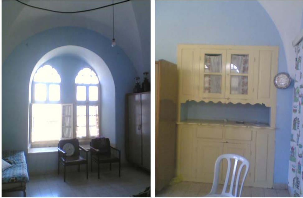
Figure 8.8: space 1.6, on the left looking west, on the right looking east
