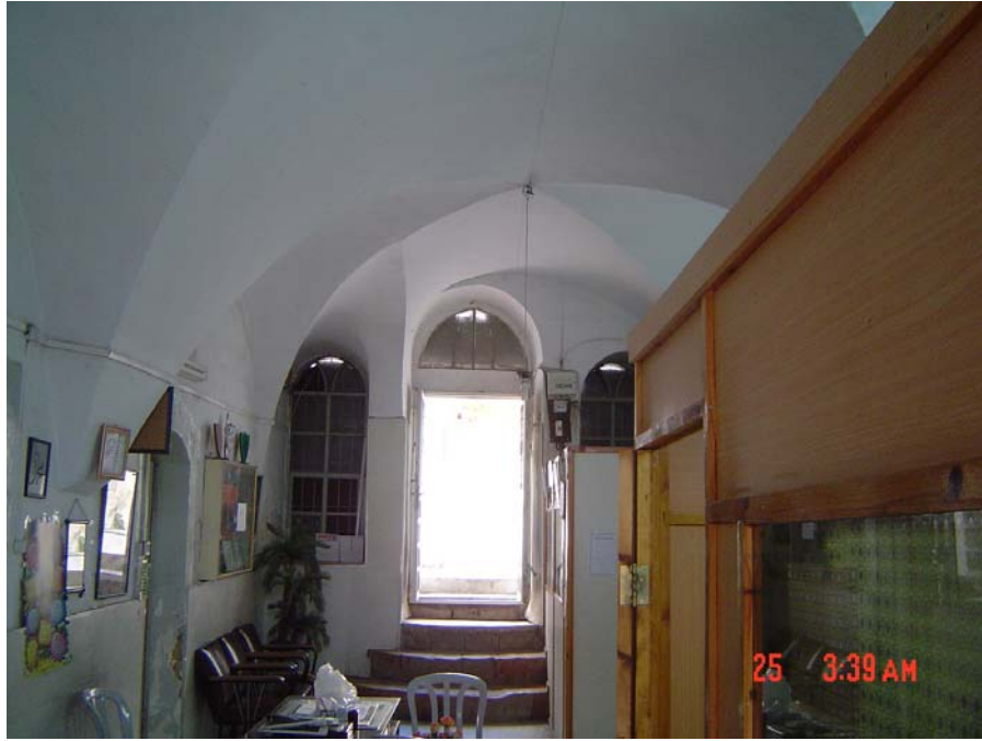
Figure 4.5: space 0.1, north wall
