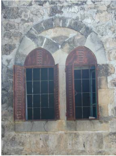
Figure 68: the south elevation left side at the upper level
