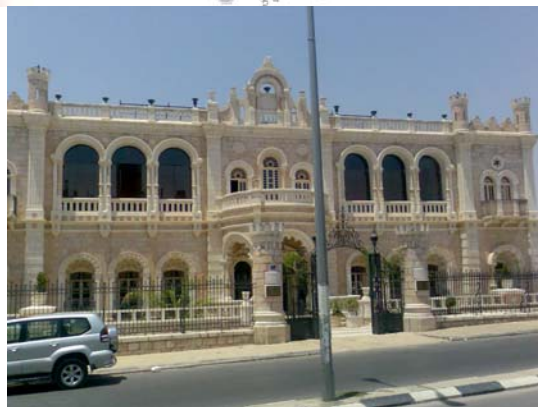
Figure 114: Jaser palace - Bethlehem constructed in 1914. Plan and main elevation Source: Khasawneh, D. (2001) Memories engraved in stone Palestinian urban mansions, Riwaq publications, Ramallah; 24
