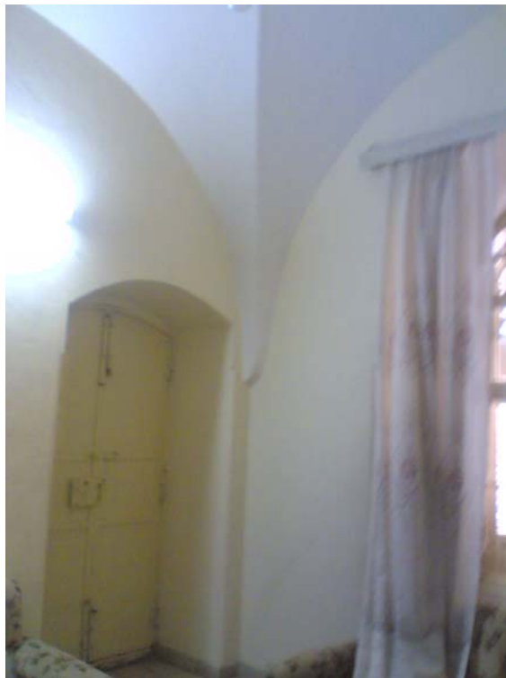
Figure 8.10: space 1.3, looking south then looking north-east corner
