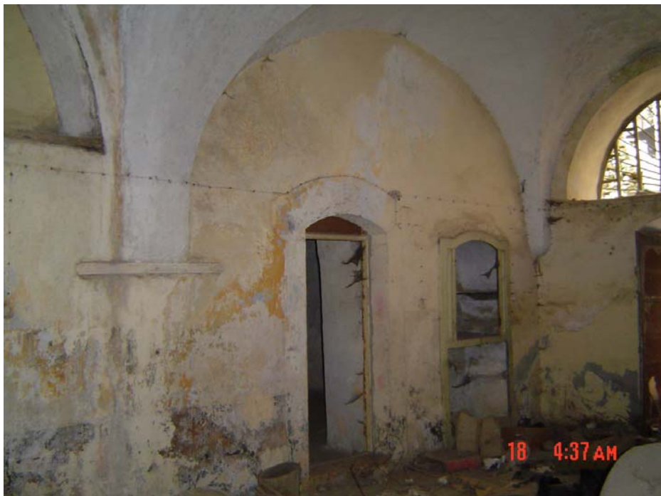
Figure 1.7: space 1.1, north wall
