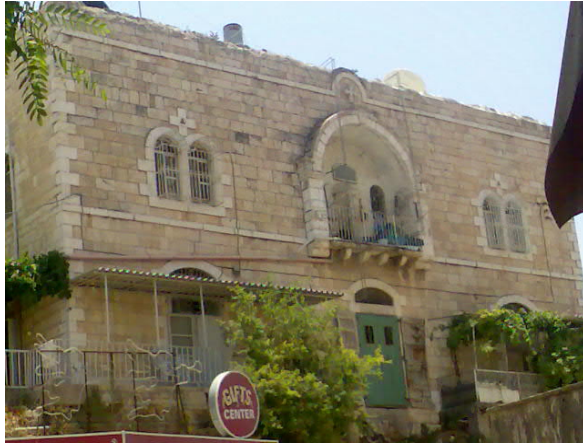
Figure 118: Central-hall house – Bethlehem, El mahed street
