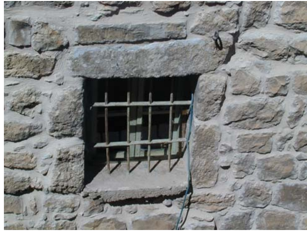
Figure 69: street level window at the south-elevation.
