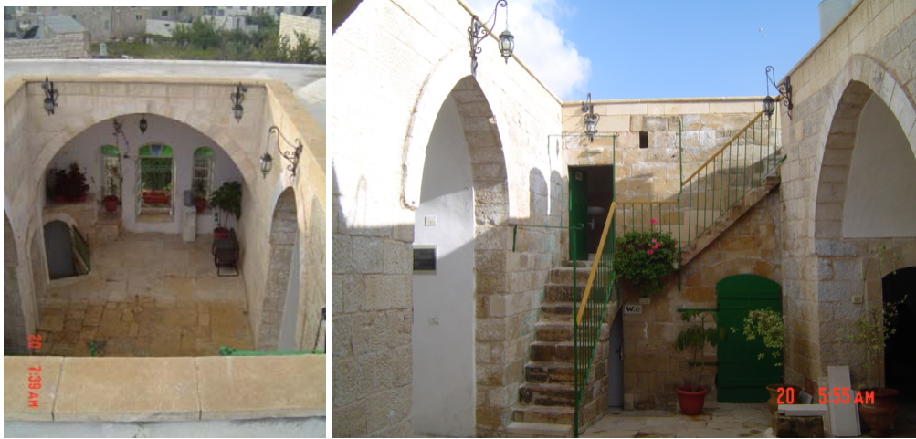
Figure 19.9: space 2.1 (Aywān ) looking west, then looking east
