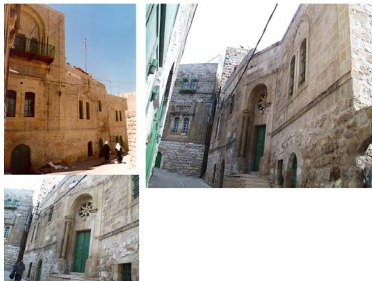
Figure 77: al-Kaliah neighborhood, al-Ja'abari house
