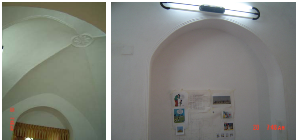
Figure 19.4: space 1.6, cross vault then north wall niche
