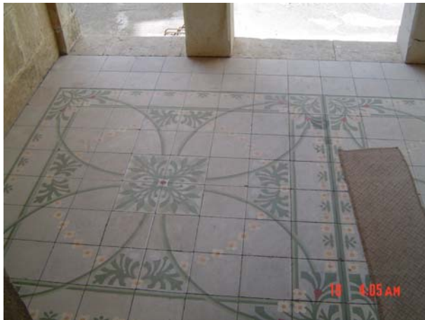
Figure 5.2: Entrance floor finish
