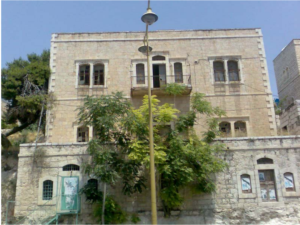
Figure 116: Central-hall house – Bethlehem, El mahed street
