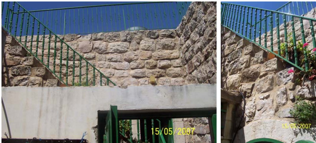
Figure 18.7: space (2.1), looking to stairs at north wall
