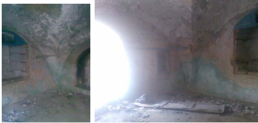
Figure 14.5: space 0.4, on the left looking south-east corner then north-east corner
