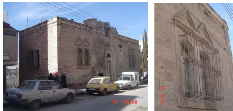
Figure 74: main (east) elevation, kaysi house Jerusalem street
