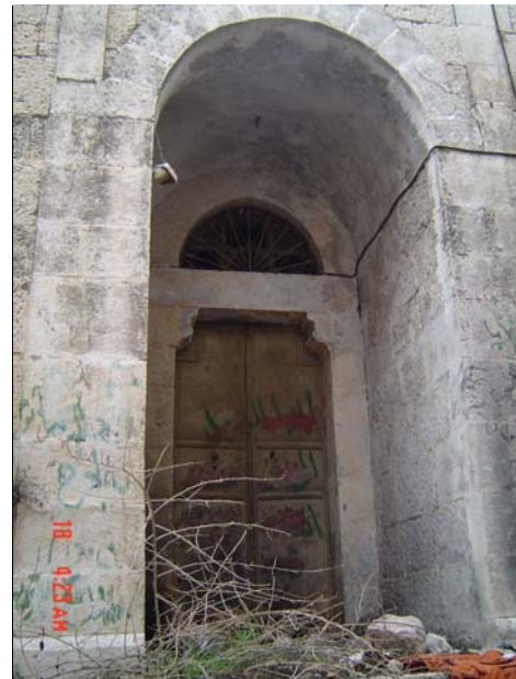
Figure 1.5: entrance on south elevation
