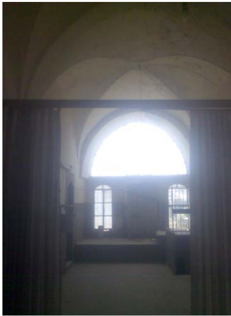
Figure 13.4: space 1.1, looking south
