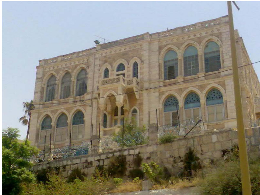
Figure 117: Central-hall house – Bethlehem, El mahed street
