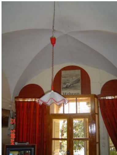
Figure 3.7: space 0.1, east wall corner
