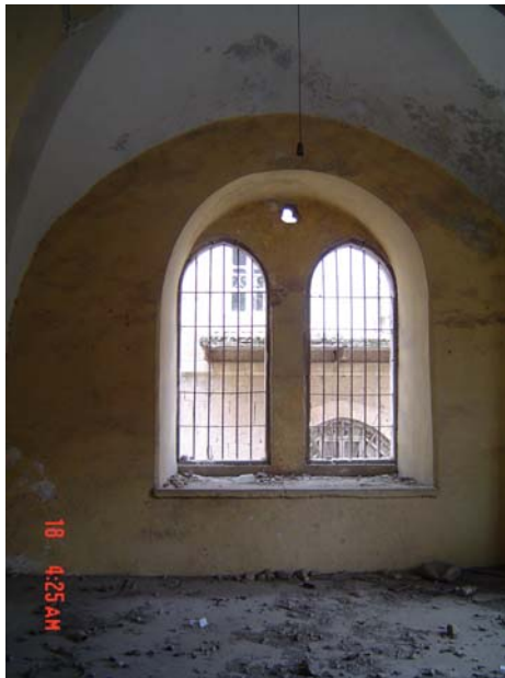
Figure 1.4: space 1.2, north wall
