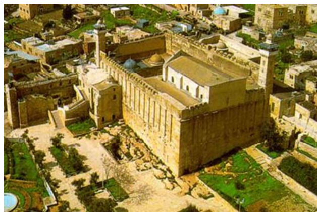
Figure 71: the Ibrahimiyy Sanctuary Source: HRC archive
