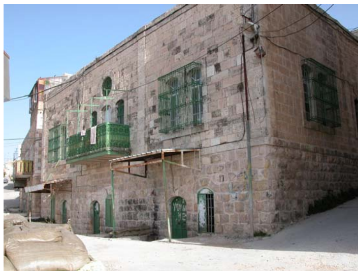
Figure 73: main (south) elevation, shohada street central-hall house
