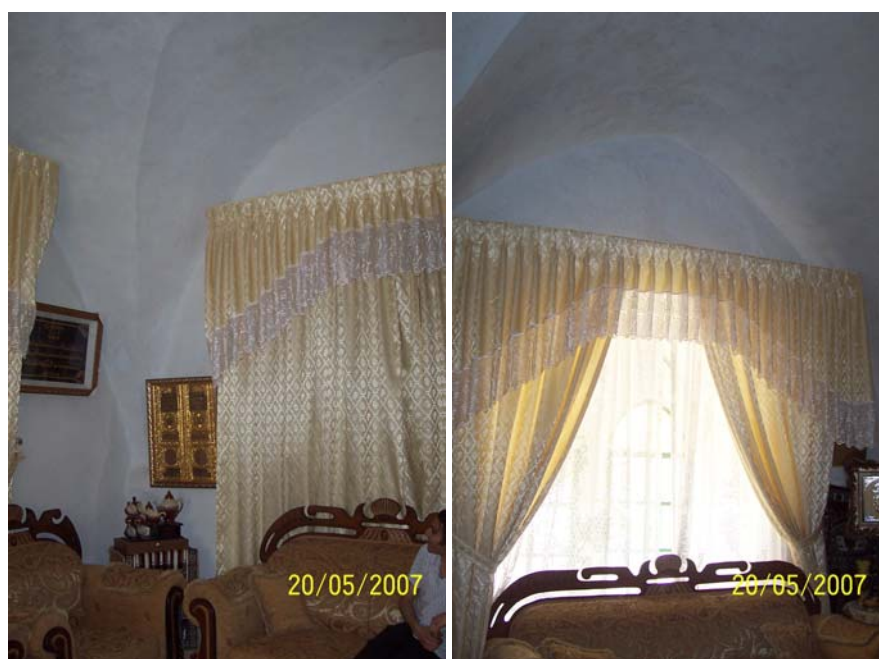
Figure 17.4: space 1.2, on the left looking south-east corner, on the right looking south wall
