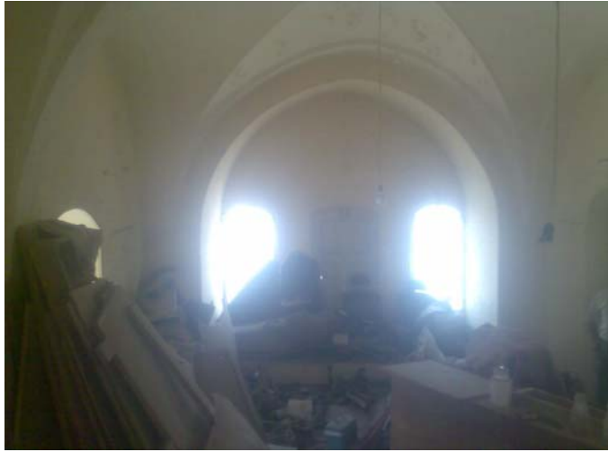
Figure 13.6: space 1.2, looking south
