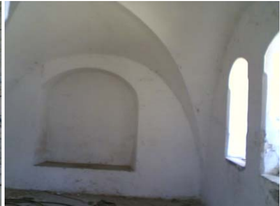
Figure 16.5: space 1.3, south-east corner
