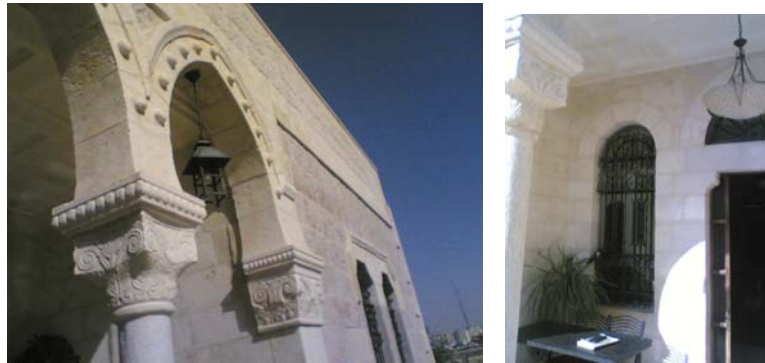
Figure 12.2: Main Elevation (West), the three arched details
