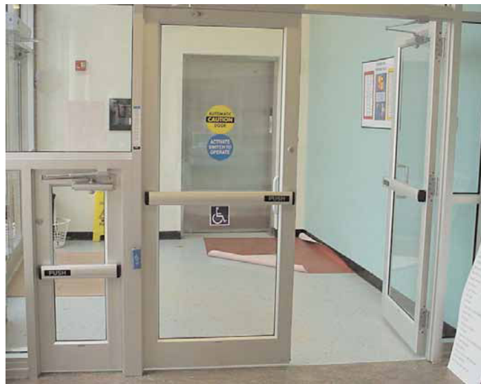
Figure 4.35. Entrances or exits which prevent uncertainty in the building. City of New York Department of Design and Construction and The Mayor’s Office for People with Disabilities. “Universal Design New York 2”. Edited by Danise Levine. Center for Inclusive Design & Environmental Access (IDEA), University at Buffalo, The State University of New York, 2003, pg. 52.
