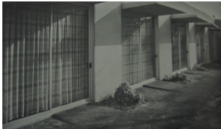
Figure 4.34. Sliding windows provide flexible use of outdoor as well as easy access to outdoors. Texas Institute for Rehabilitation and Research. “Hospitals, Clinics, and Health Centers”. New York: F. W. Dodge Corporation, 1960, pg. 200.
