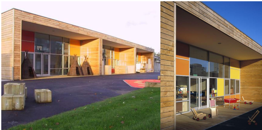
Figure 4.26. Inclusive playgrounds for children as extensions of indoor spaces. Broadwater Farm Children's Centre designed by Gollifer Langston Architects who gets the RIBA Inclusive Design Award in 2007. Retrieved on November 27, 2008 from http://www.architecture.com/Awards/RIBAAwards/Winners2007/London/Broadwater/BroadwaterFarmChildrensCentre.aspx
