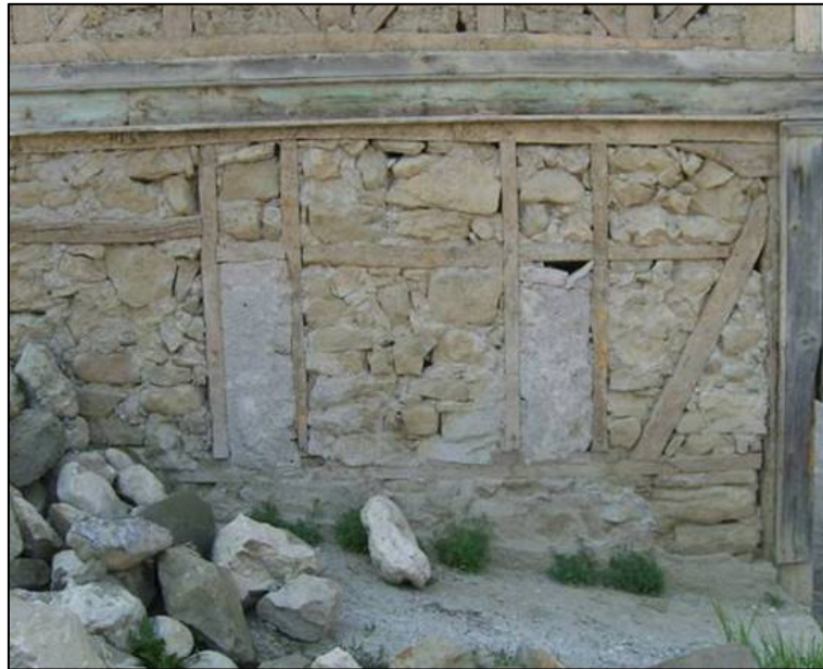
Figure 4.18. Timber skeleton with stone infill on Çakırlar Konağı (author, May 2007)
