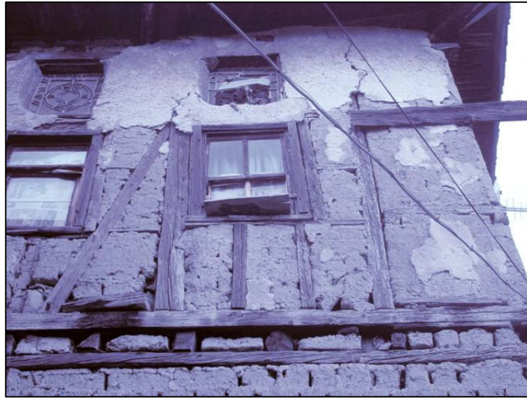
Figure 4.14. Floor joists visible on exterior façade of parcel 664 (author, May 2007)
