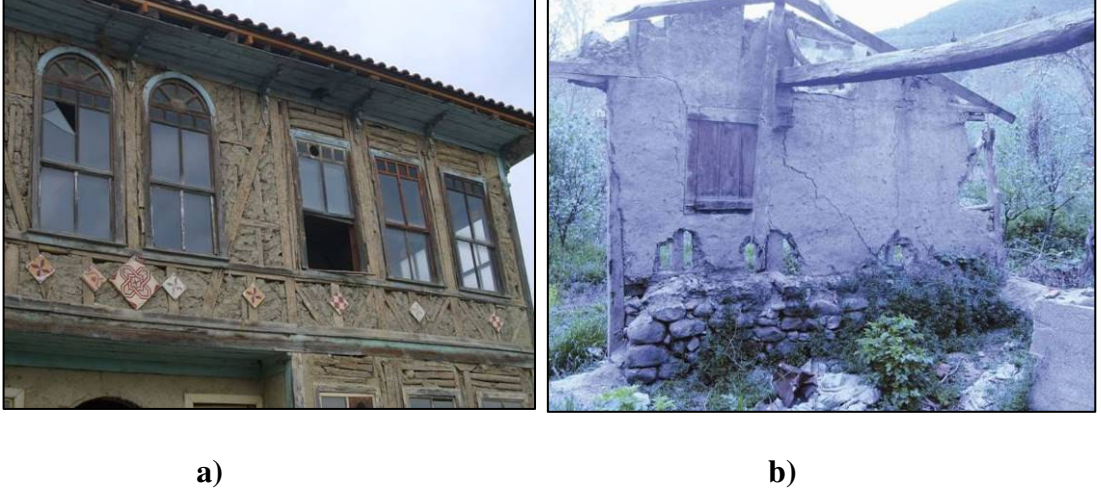
Figure 4.10. Timber skeleton construction with mudbrick infill, a) Front façade of Çakırlar Konağı (author, May 2007), b) Standing wall of sheet 6, parcel 702 (author, May 2007)
