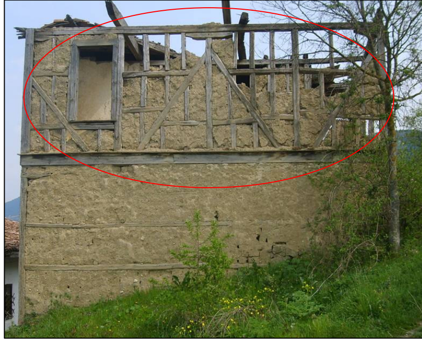
Figure 4.11. Timber framed construction of Hisar Evi (author, May 2007)
