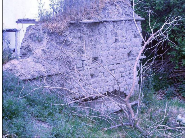
Figure 4.6. Masonry mudbrick construction in Great Mosque District (author, May 2007)
