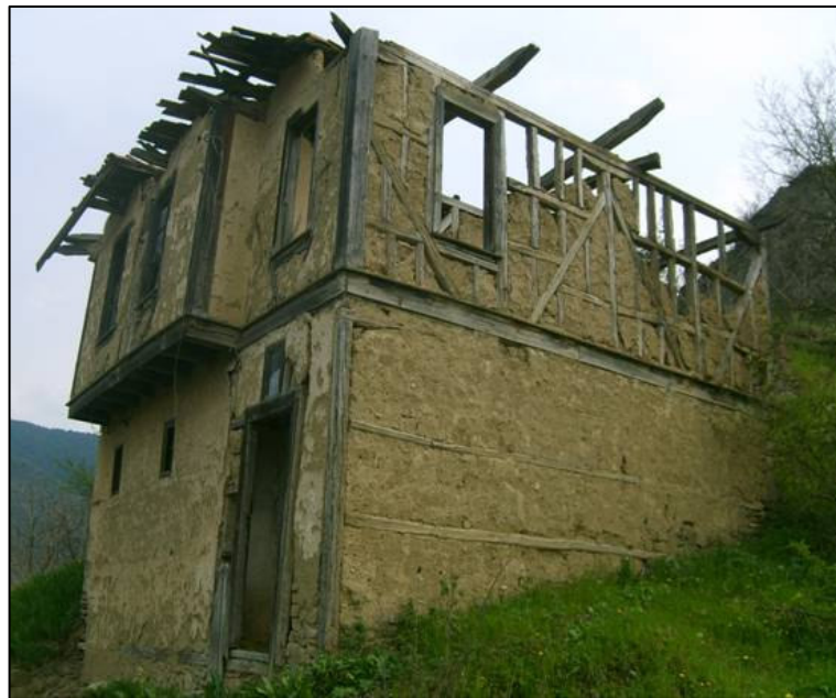
Figure 4.22. Masonry mudbrick with corner posts at Hisar Evi (author, May 2007)
