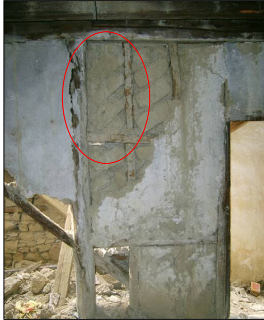
Figure 4.15. Mudbrick inserted a bit slanted in order to increase the stability of the structure-Hisar Evi (author, May 2007)
