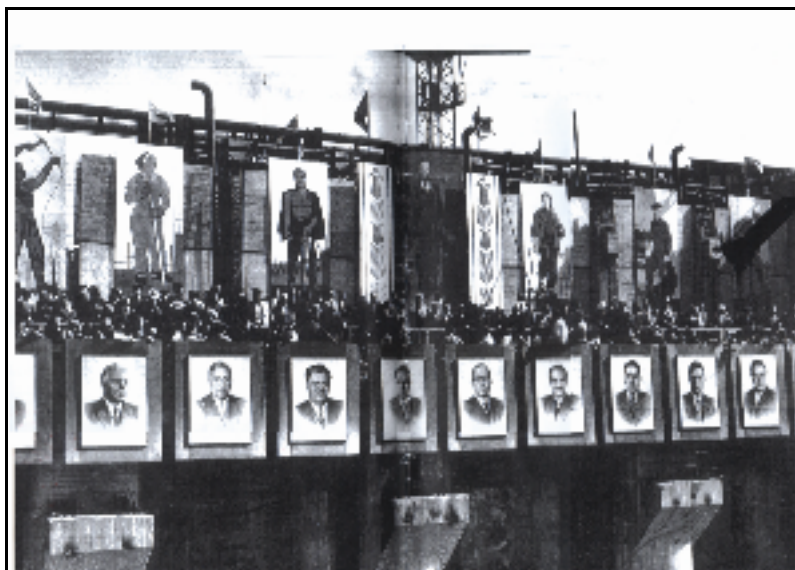
Figure 25: Niels Gutschow, "Happiness in the Light. The Construction of a New Power Plant in Kaunas, Lithuania, 1959." in Cor Wagenaar (ed.), Happy. Cities and Public Happiness in Post-War Europe , Rotterdam: NAI Publishers, 2004, pp.92-93.
