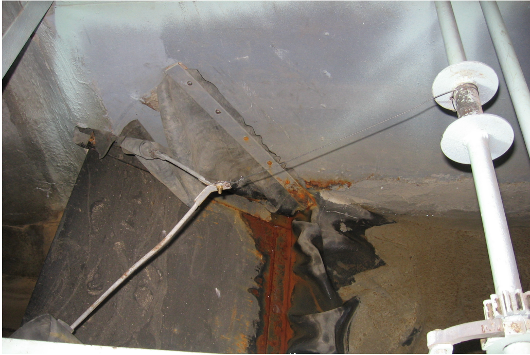
Figure B.4 Flap gate installed at downstream
