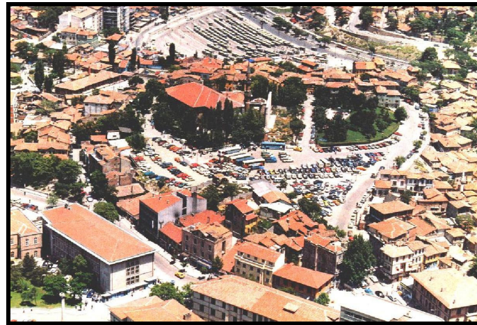
Figure 4. 33 Hacibayram Square before uncompleted implementation (Source: Mehmet Tunçer).
