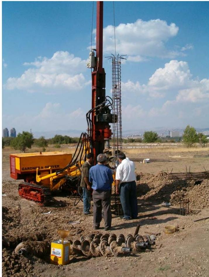
Figure 3.1 Construction of bored piles
