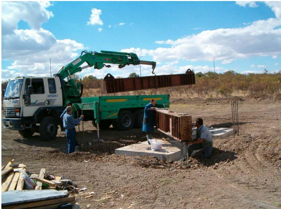
Figure 3.4 Replacement of steel reaction beams
