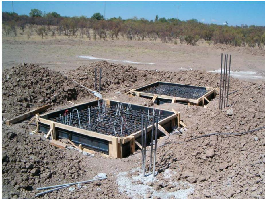
Figure 3.3 Construction of model piled raft
