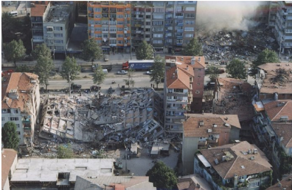
Figure 1. 3 General building damage in the vicinity of Gölcük. Source: http://www.eas.slu.edu/Earthquake_Center/TURKEY/xx3.jpg
