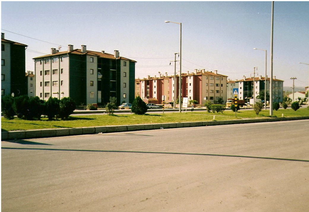
Figure 3. 9 Post-earthquake apartment buildings in Afyon after 1995 Dinar Earthquake.
