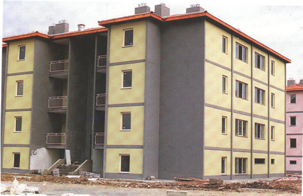
Figure 3. 8 A post-earthquake apartment building in Erzincan after the 1992 Erzincan Earthquake.
