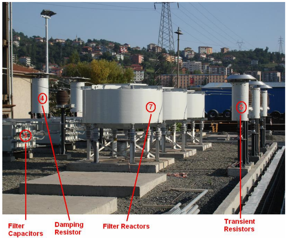
Figure 3.3. Views of power system elements of SVC (outside)
