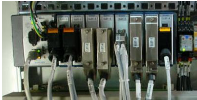
Figure 3.15. NI cRIO mounted inside the control enclosure
