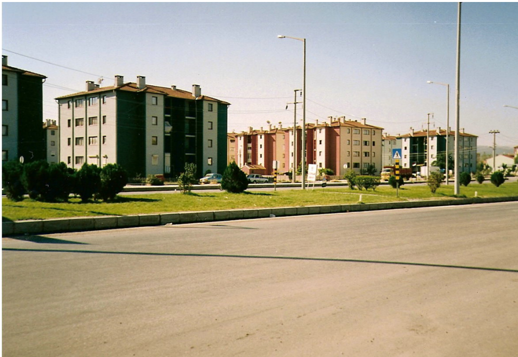
Figure 3. 9 Post-earthquake apartment buildings in Afyon after 1995 Dinar Earthquake.
