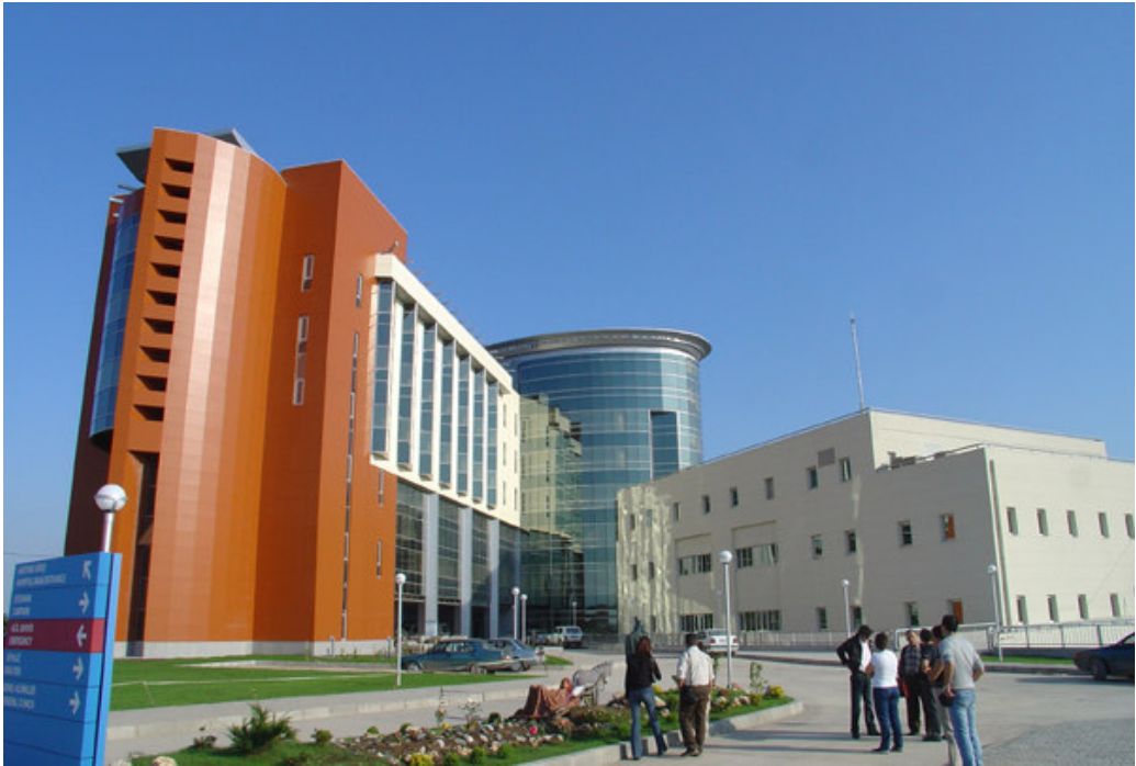
Figure 6. 5 SSK Adapazarı Hospital as built. (Cem Altınöz, Önder Kaya, Enis Öncüoğlu, 2004)
