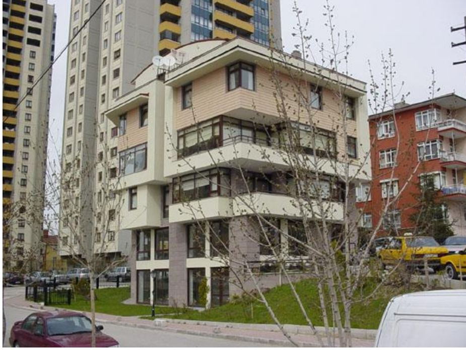
Figure 6. 15 An apartment building in Dikmen Ankara. (Tamer Başbuğ, Baran İdil, Hasan Özbay, 2001) Source: http://arkiv.arkitera.com/p2960-dikmende-apartman.html
