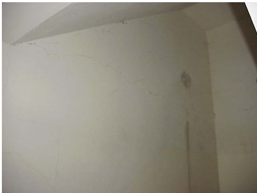
Figure 3.8 : Horizontal cracks on the northern flange of shear wall P1, at the slab level
