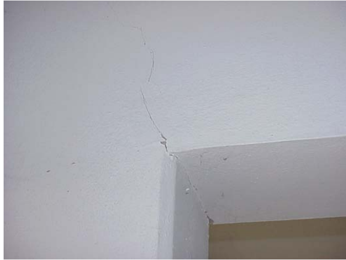
Figure 3.5 : Flexural crack at the end of beam K154, where it spans into the column S04
