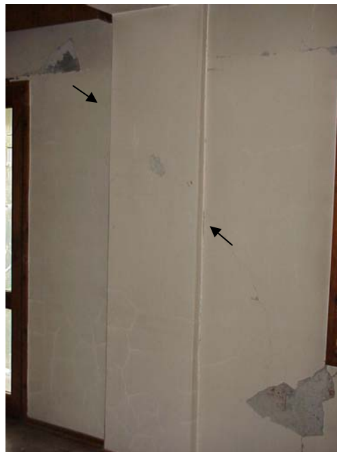
Figure 3.6 : Diagonal crack passing through beam K131, column S6 and the adjacent walls, at the first story
