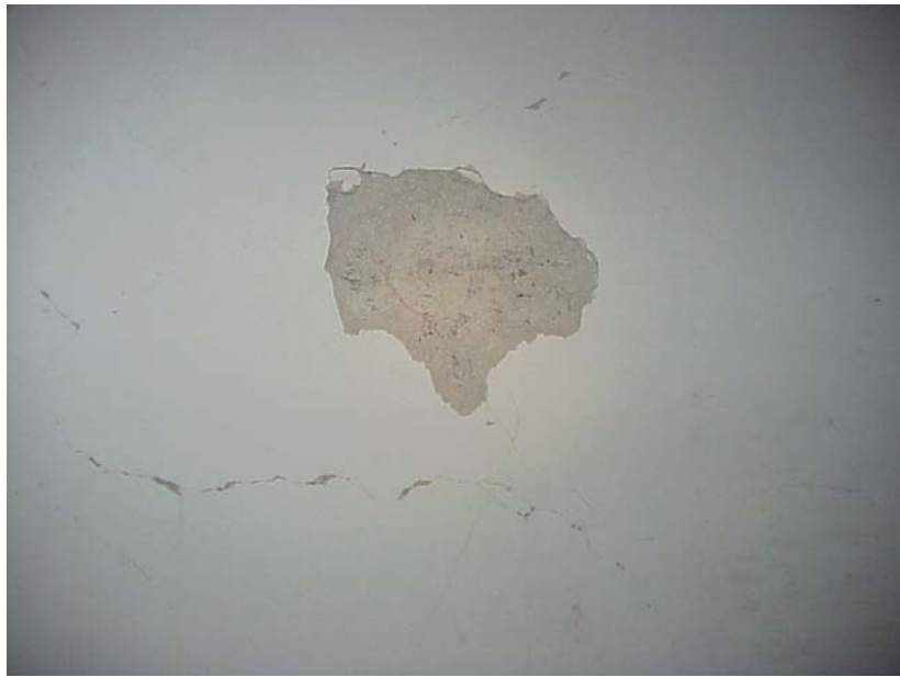
Figure 3.7 : Diagonal cracks on the web portion of shear wall P1 indicating southward movement
