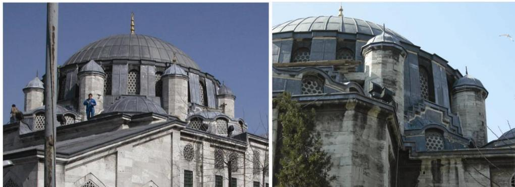
**Figure 37** The dome of the Azapkapı Mosque and eight weight turrets around it. Photographs by C. Katipoglu, 2006.
