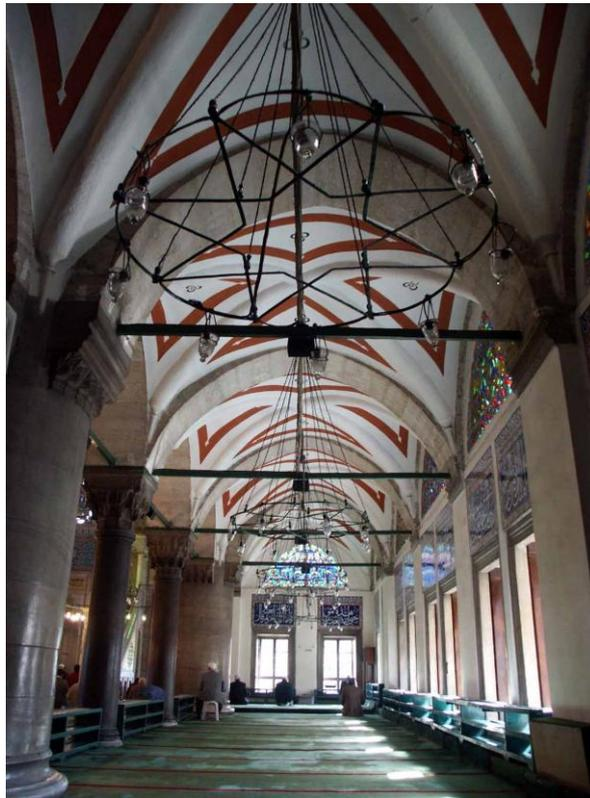
**Figure 109** The cross-vaulted side galleries of the Kılıç Ali Pasha Mosque. Photograph by C. Katipoğlu, 2006.
