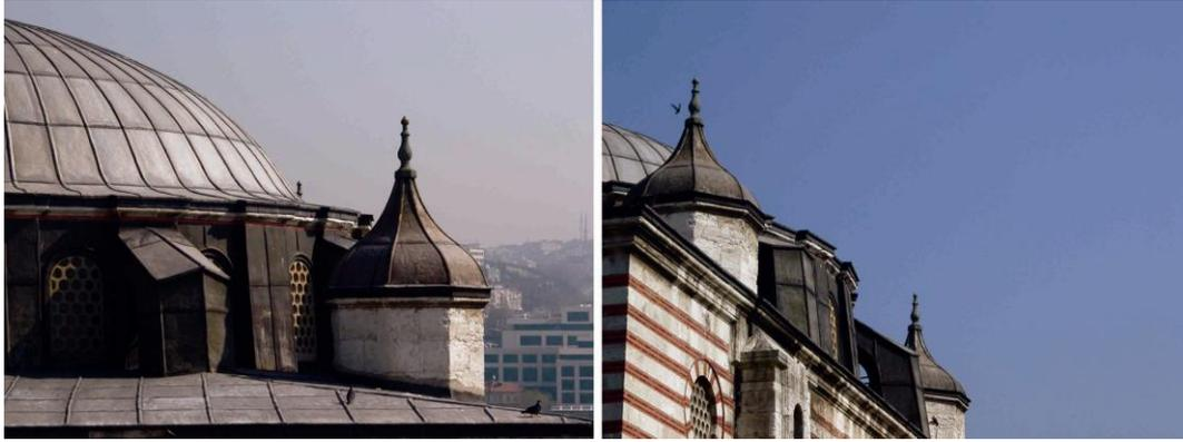
**Figure 137** The weight turrets covered with onion domes emphasized the appearance of the main dome. Photographs by C. Katipoğlu, 2006
