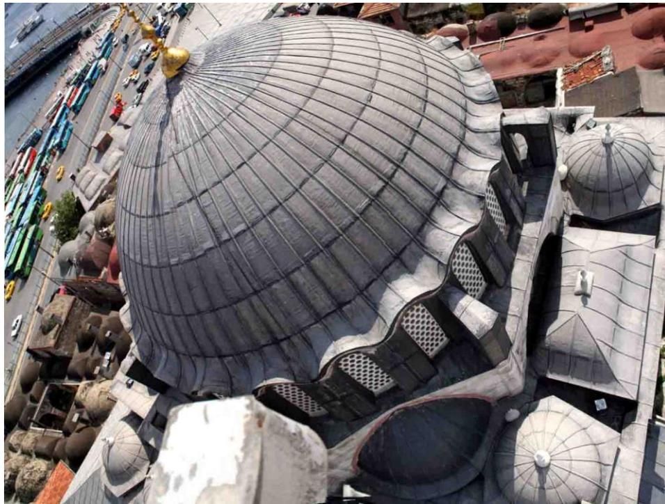
**Figure 17** One vault and two dome cover of the west wings of the mosque. Photograph by C. Katipoğlu, 2006.
