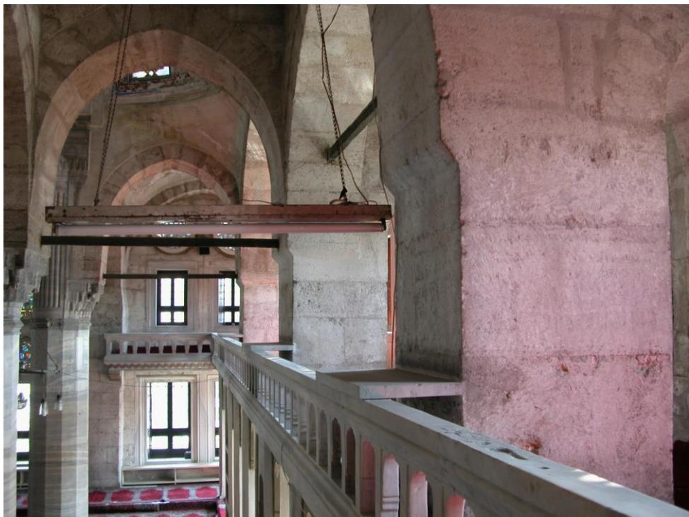
**Figure 42** The arches of the Azapkapı Mosque which tie to the buttresses and pillars. Photograph by C. Katipoglu, 2006.
