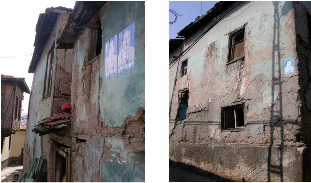
Figure 2.1 General views of Eylül Lane House
