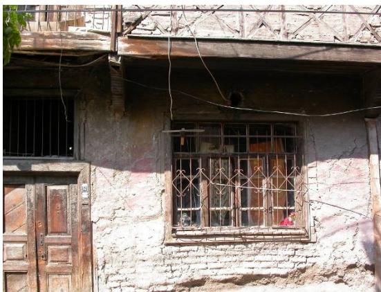
Figure 2.4 General view of Öksüzler Lane House
