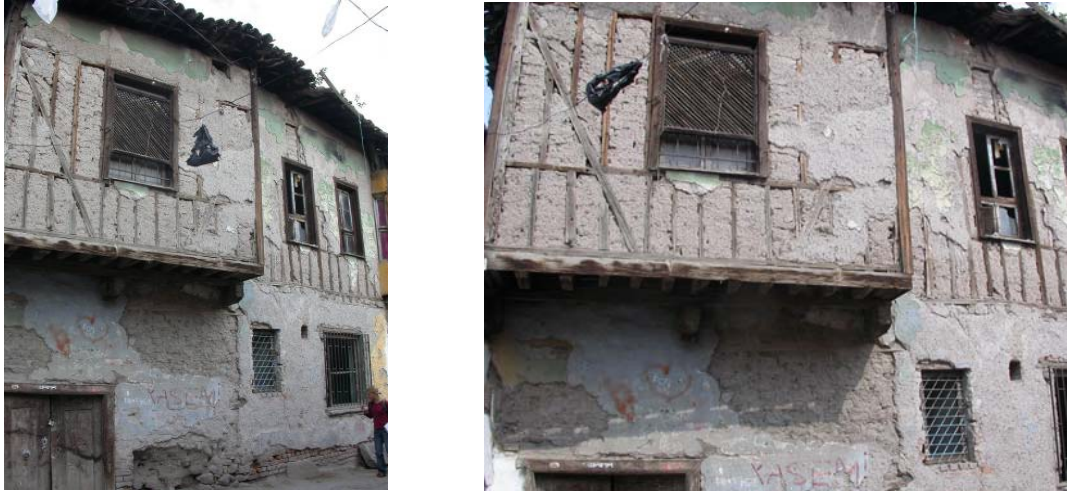
Figure 2.3 General views of Yeniıldırımlar Lane House
