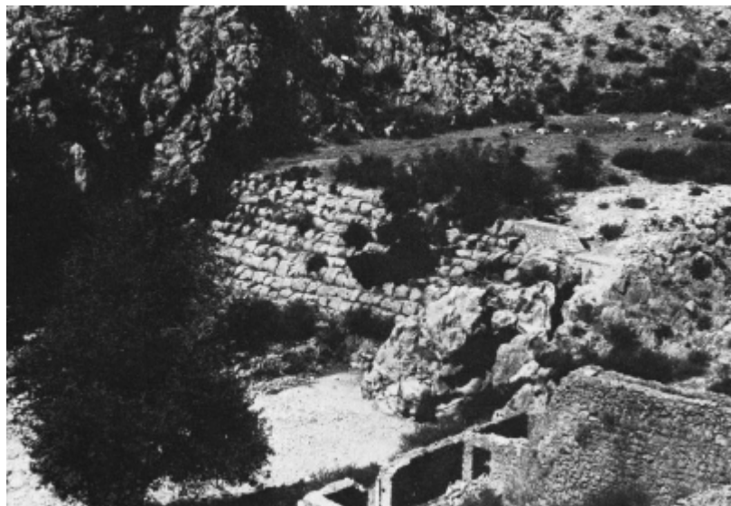
Figure 9: Mytikas Valley Dam from East (Murray 1984: Plate 32)
