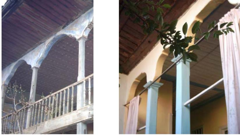
**Figure 132, Timber colonnades with Bursa-type arches in *hayats* of a demolished dwelling and Case 1 (Taşdöğen)**
