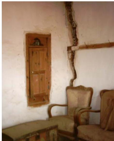
Figure 62, Case 3, Crack on the wall of a room upstairs (Taşdöğen)
