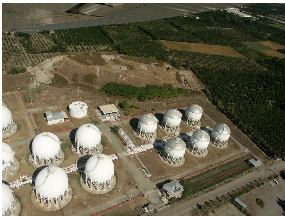
Fig 2.2: Aerial view of the site from West, with BP propane gas tanks in foreground (Photo: M.-H.Gates).
