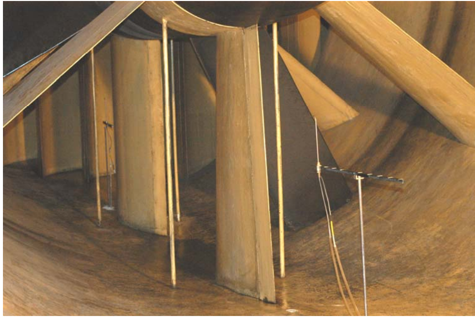
Figure 3.7 Test Picture (Up and Downstream of the Fan).
