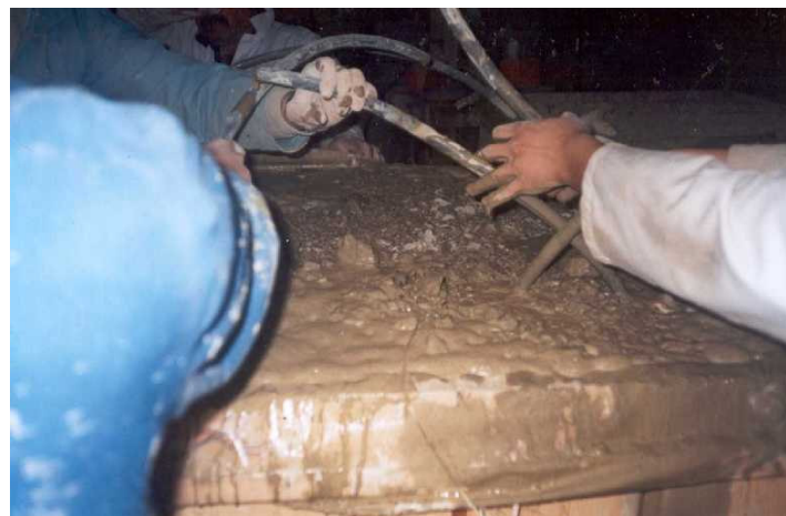
Figure 3.16. The alternating pumping of the five insert pipes
