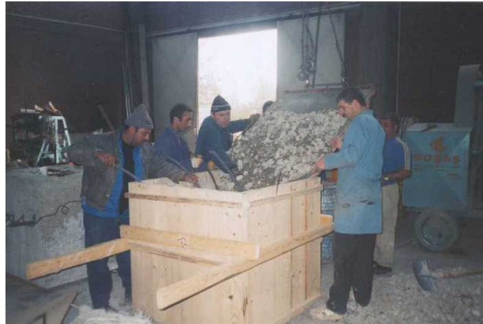
Figure 3.5. The preplacing of coarse aggregates into the formwork
