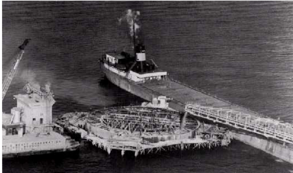
Figure 2.11. The coarse aggregate was placed from the self-unloading boat seen on the right into the pier form seen at the middle and then grouted by the semi-automatic plant seen on the left during the construction of Mackinac Bridge
