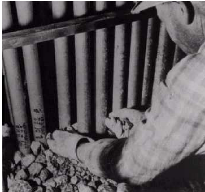
Figure 2.1. Preplacing of heavyweight coarse aggregate (barite) by hand during the construction of a biological shield at Materials Testing Reactor (Arco, Idaho)
