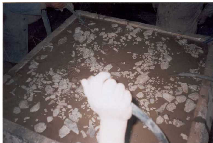
Figure 3.6. The grout is pumped through the insert pipes till it rises upto the top surface of the preplaced coarse aggregate mass
