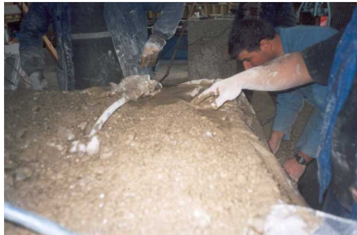
Figure 3.12. The connection of the pump outlet and the insert pipe
