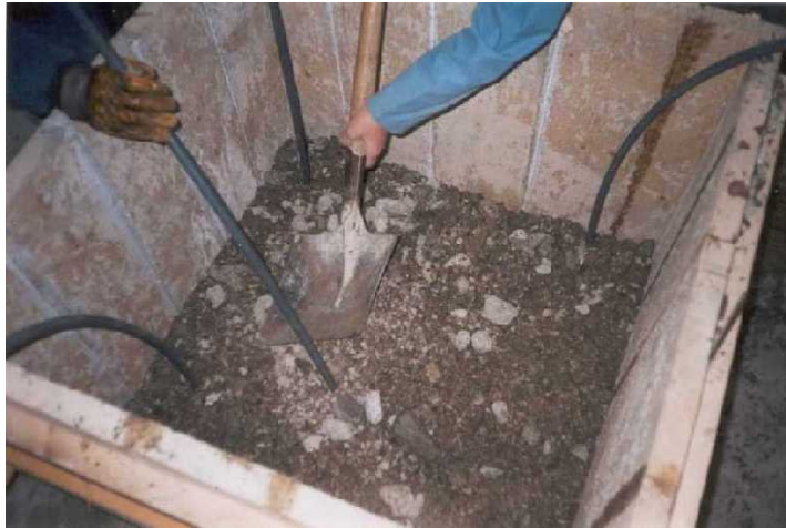
Figure 3.15. Locating of the insert pipes during the placement of aggregates
