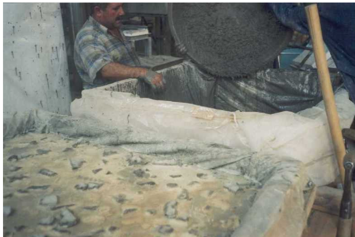
Figure 3.7. The self-compacting mortar is just poured over the preplaced coarse aggregate without applying any injection
