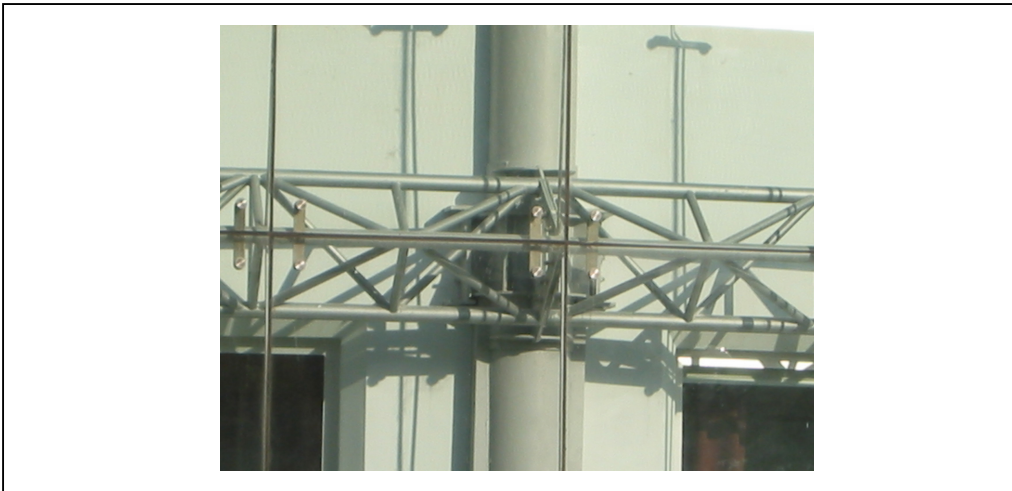
Figure 4.30. The space framed truss hinged to the column. Source: By author, 2003
