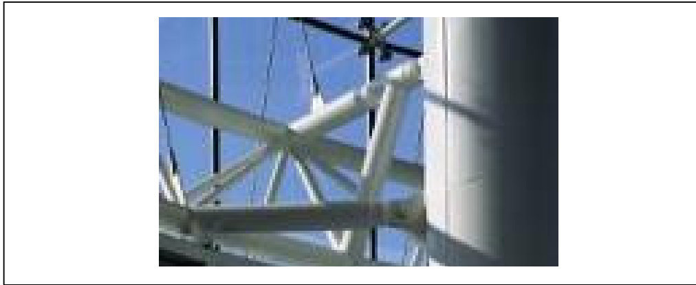
Figure 4.35. Hinged support Source: www.mero.de , 2003
