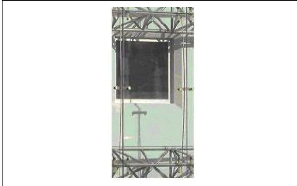
Figure 4.36. A glass pane with 6 holes. Source: By author, 2003
