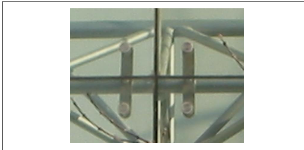
Figure 4.37. Two armed post mounted spiders of the façade
