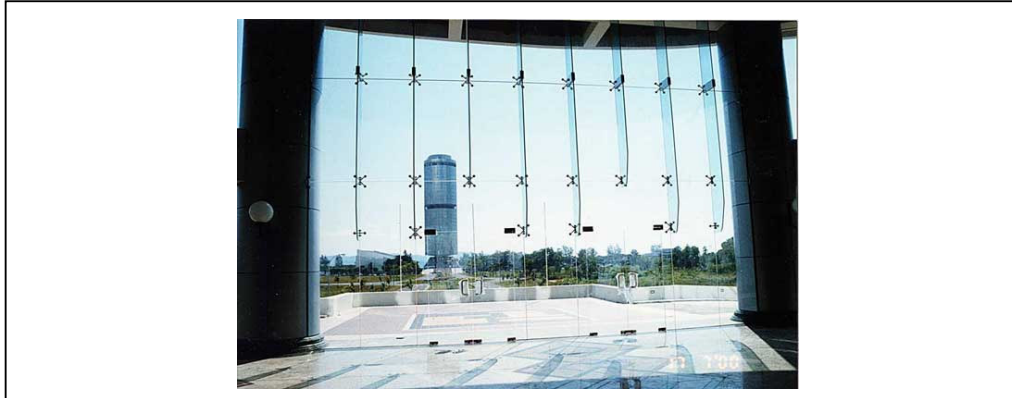
Figure 4.15. Glass Fin System. Source: C.R.Laurance Co.Inc, 2003
