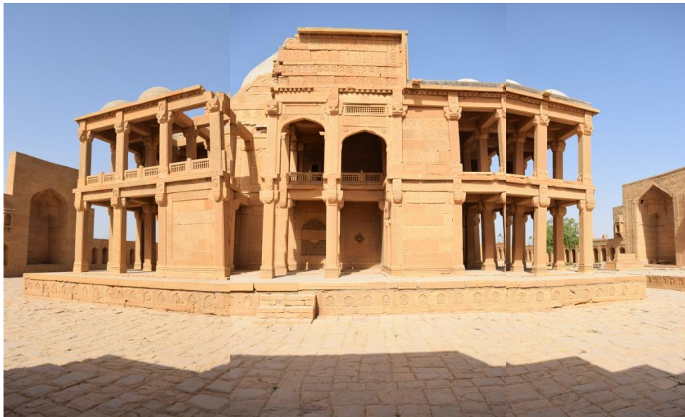
Figure 47: East elevation with colonnaded terrace and barely visible dome of the tomb chamber behind with flanking north and south iwans of the enclosure, Tomb of Isa Khan Tarkhan II.
