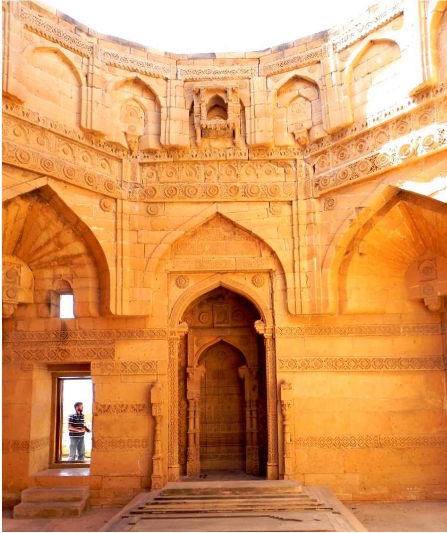
Figure 20: Interior with triple mihrab, and zone of transition, Tomb of Jam Nizam.
