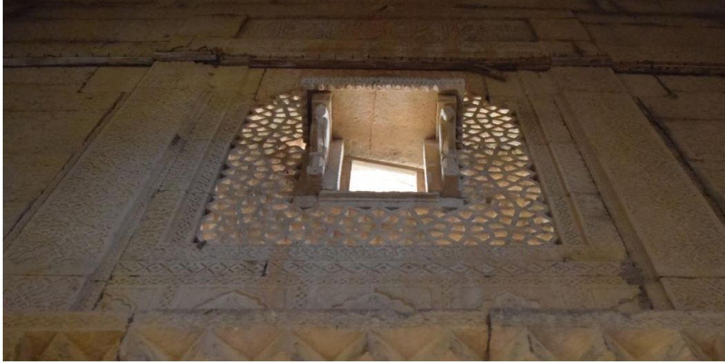
Figure 58: Miniature oriel in the interior perched in the middle of pointed arched opening with a stone screen having six pointed star geometric grid pattern, Tomb of Isa Khan Tarkhan II.
