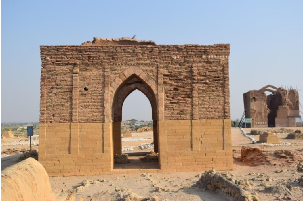
Figure 68: South elevation with dentil moldings and vertical linings, Tomb of Malik Rajbal (1457 CE), Samma Period.
