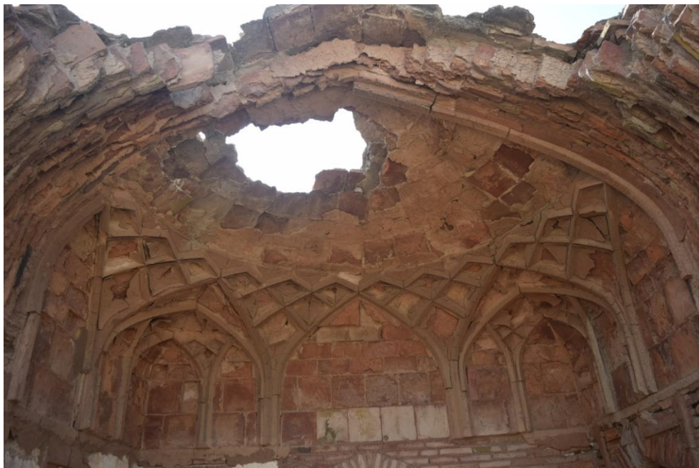
Figure 82: Unknown brick tomb with stalactite interlacement is lined with stucco moldings, Arghun / Tarkhan Period.
