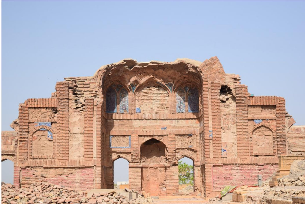
Figure 83: Unknown brick enclosure with stalactite interlacement achieved through crisp brick linings opposed to stucco and adorned with blue tile work, Tarkhan/ Mughal Period.
