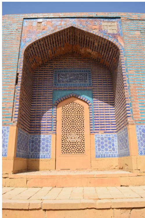
Figure 78: Eastern façade with stone, skirting corner pilasters and geometric screen, Tomb of Jani and Ghazi Beg.
