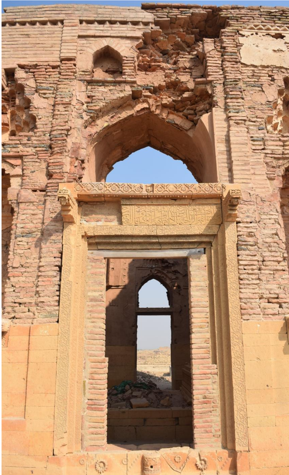
Figure 73: Southern opening with stone carving details, carved moonstone threshold and brick the moldings above, Kaus Sultani.
