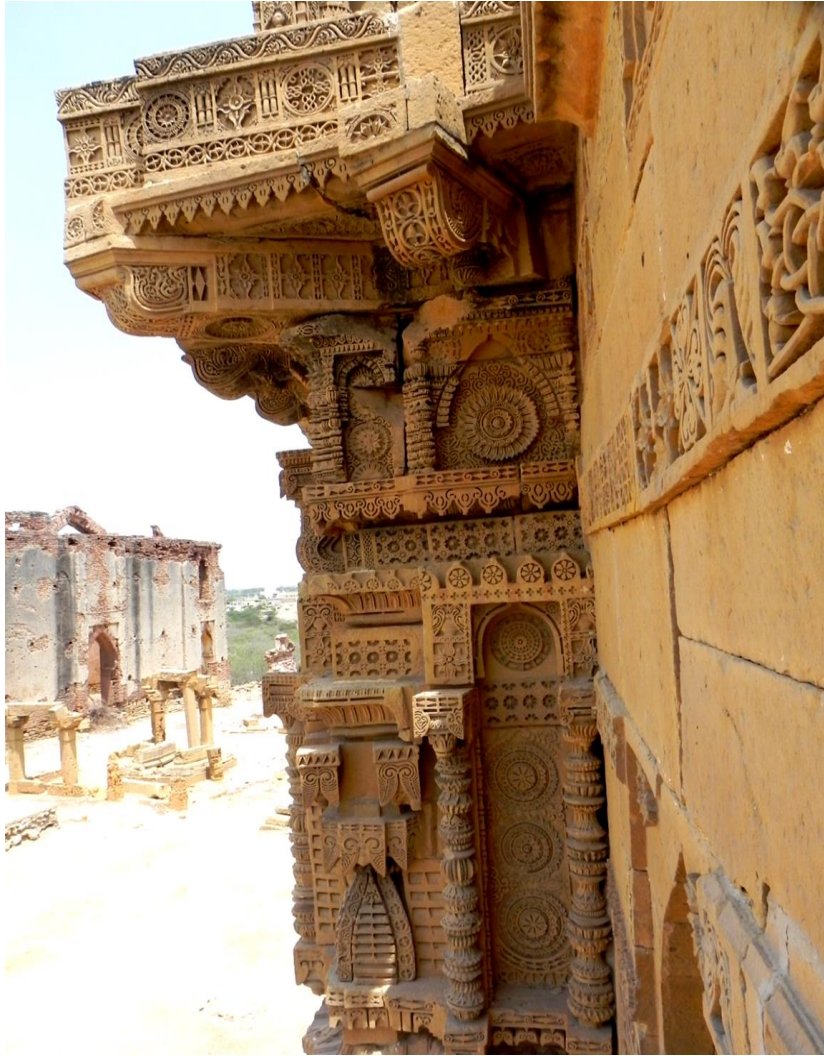
Figure 19: Third level of projecting balcony showing the winding brackets and miniature sikhara , Tomb of Jam Nizam.
