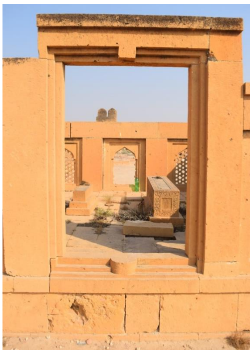
Figure 64: Non ornate variety of moonstone step at the threshold, unknown enclosure with tracery/ jali pattern – Arghun period.
