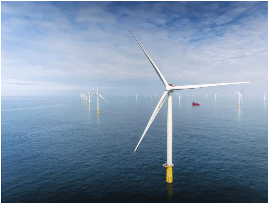
Figure 4.4. Offshore Wind Farm (Fard, 2018)
