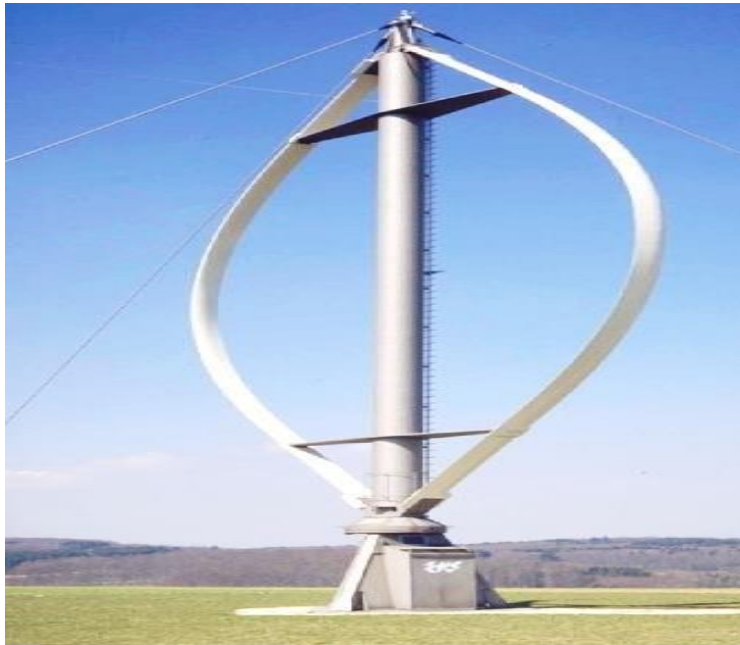
Figure 4.2. Vertical Axis Wind Turbine (Aboufaires, 2015)
