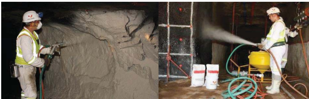
Figure 2.2 Typical Underground applications of TSLs (Ferreira and Piroddi,2012)
