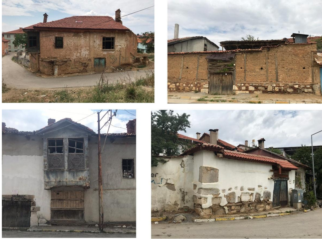
Figure 3.64. Yalvaç, Kaş District, spolia used in the construction of village houses, 2019
