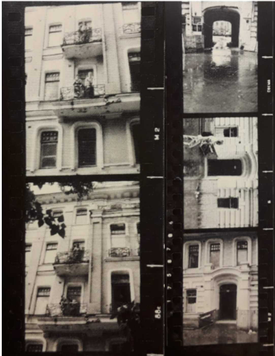
Figure 3.26. The facade and entrance of House No:18, from the stills of George Kiesewalter, 1987 Garage Museum of Contemporary Art, George Kiesewalter archive
