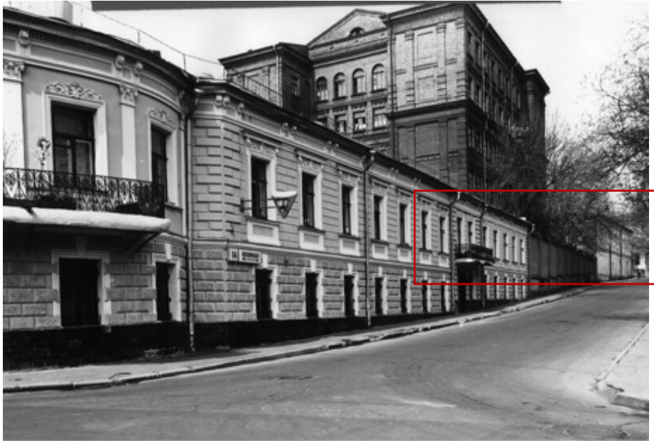
Figure 3.17. Building of “Kindergarten”, Moscow, 1970s, with the rooms of the artists marked Central State Archive of the City of Moscow” (“TsGA Moskvi”)
