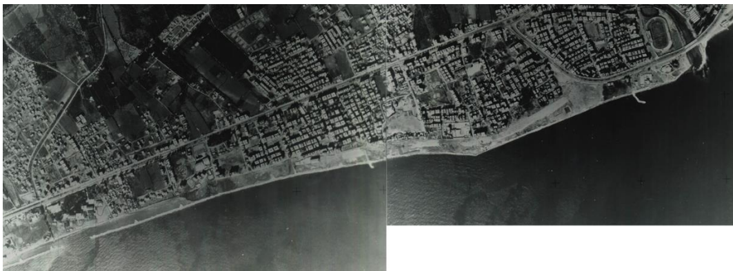
Figure 4.9. Aerial views indicating ongoing filling works between Hilton Hotel and Pozcu District in 1991 (The archive of the Metropolitan Municipality of Mersin)
