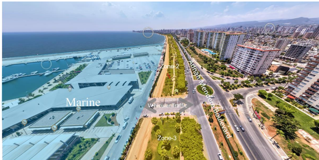
Figure 4.24. The entrance of Mersin Marine and near surrounding area (produced by the Author, Nov 2015 dated aerial view taken from vr.mersin.bel.tr)
