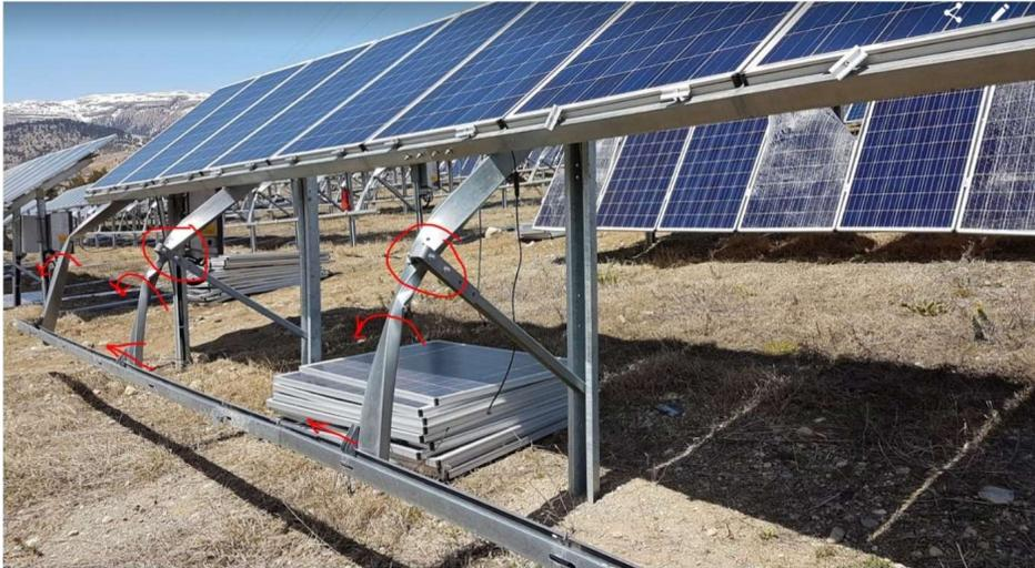
Figure 37- Damaged Main Beam-1
