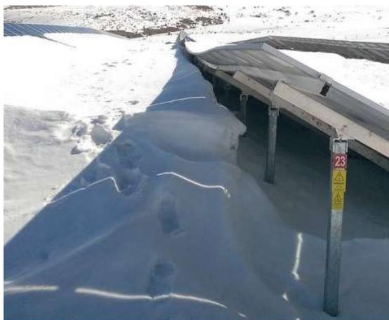
Figure 36- Snow Accumulation on PV Panels-3
