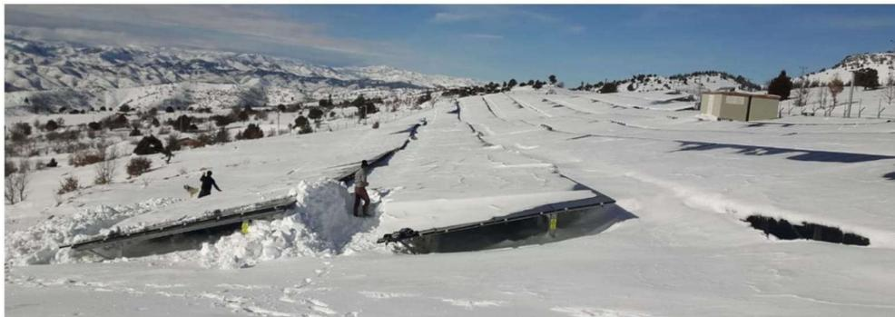
Figure 35- Snow Accumulation on PV Panels-2
