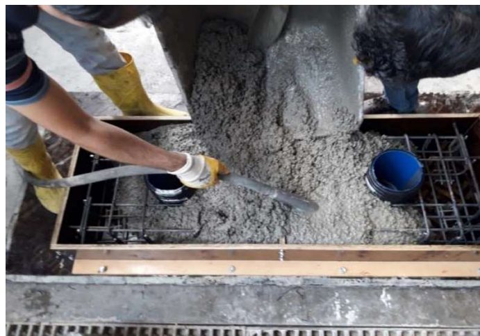
Figure 2.3. Concrete casting stage
