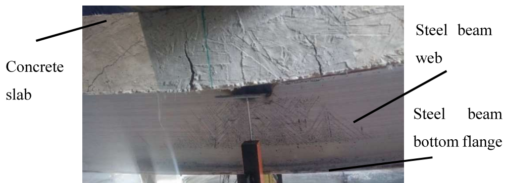
Figure 3.15. Yielding of steel section observed during bending test (Specimen-2)
