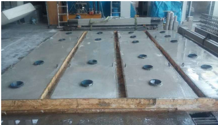
Figure 3.2. The precast deck specimens
