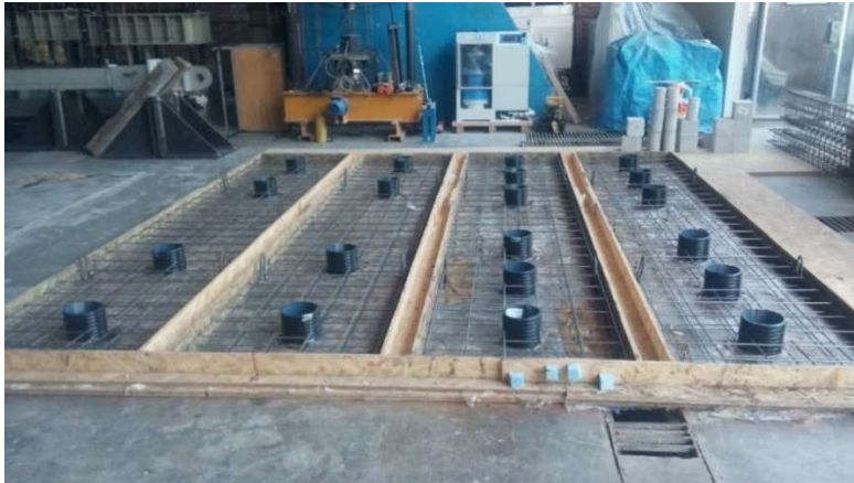
Figure 3.1. The corrugated pipes placed in formworks of beam specimens
