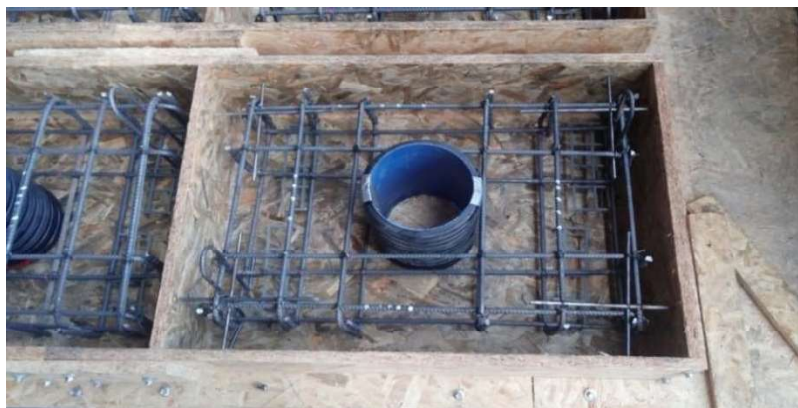
Figure 2.1. The molds with corrugated pipes and reinforcement bars
