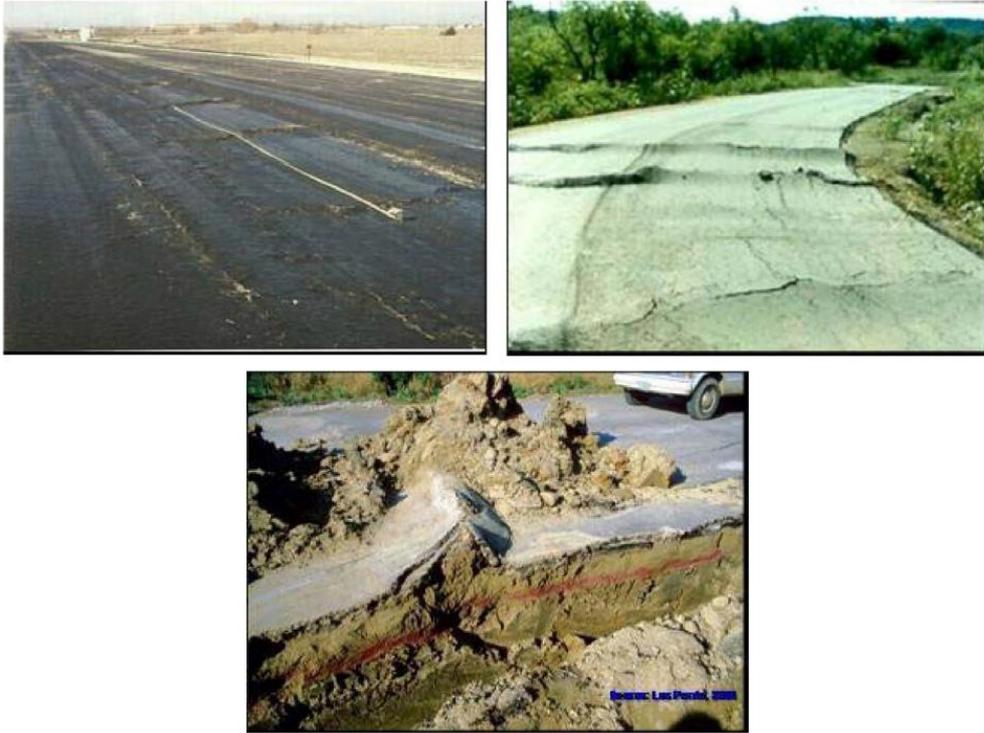
*Figure 3.1.* Vertical heave problem in roads due to the ettringite formation (Puppala et al., 2019)
