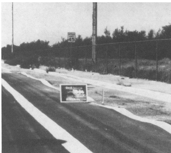
*Figure 3.6. Pavement surface failure (Mitchell, 1986)*
