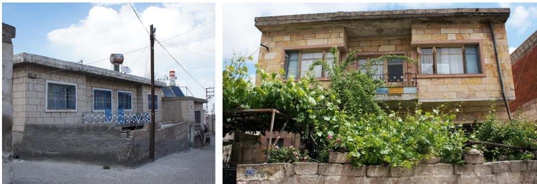
Figure 4.38. Examples for masonry walls with RC Frame slabs of new buildings
