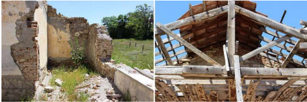
Figure 3.19. Structural techniques can be read with these photos of dormitory buildings, stone and brick masonry walls, on left, the roof construction on right (Aladağ, 2019)
