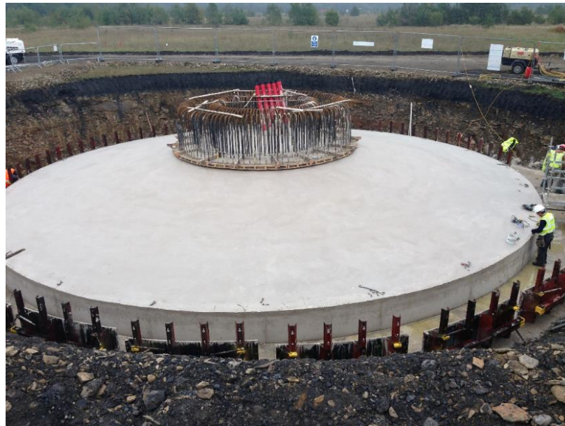
Figure 2.5. An Almost Completed Wind Turbine Gravity Base Circular Foundation. Retrieved from Partnership for Renewables (2013)
