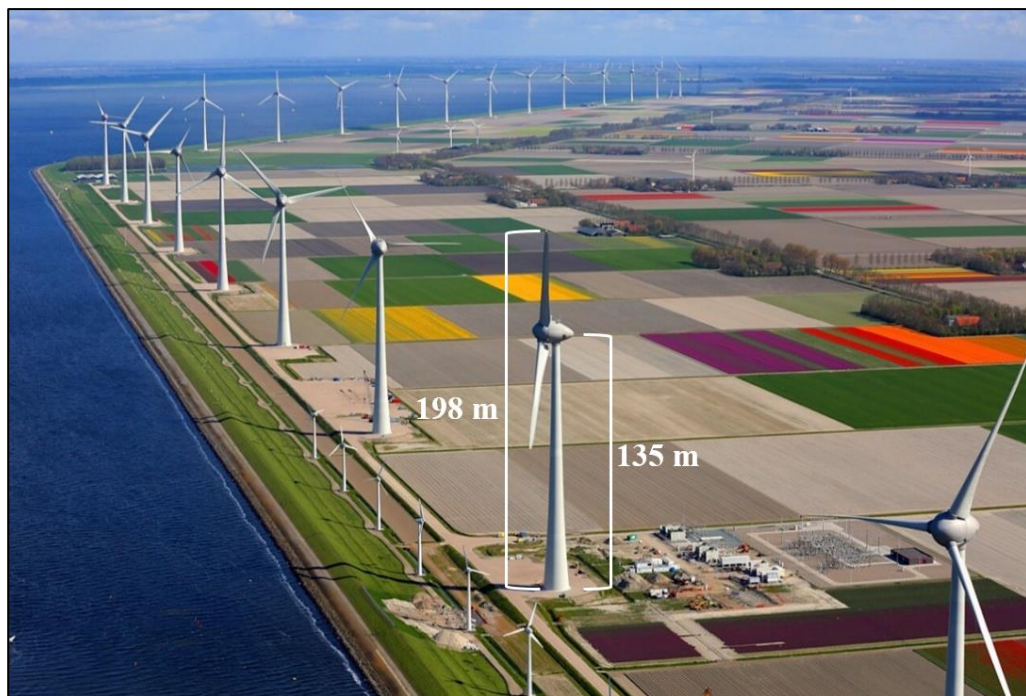
Figure 2.1. Horizontal Axis Wind Turbines with Rated Power of 7.5 MW at Noordoostpolder Windpark in the Netherlands
