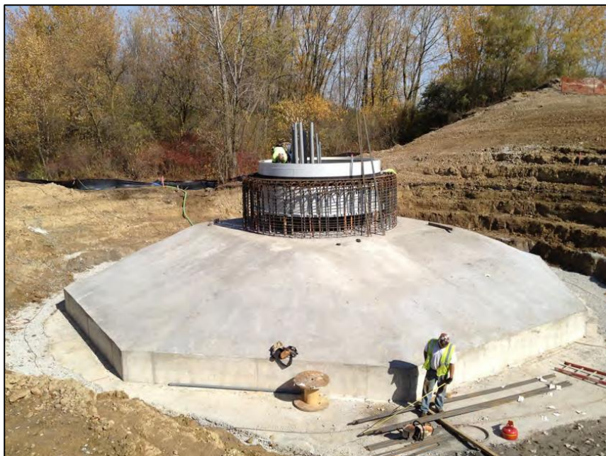
Figure 3.1. The Wind Turbine Foundation Constructed for the Project
