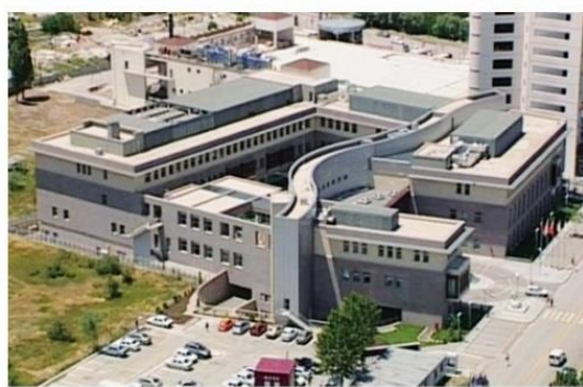
Figure 5.42. Tobb-ETU Hospital, general view, indoor, courtyard, general view
