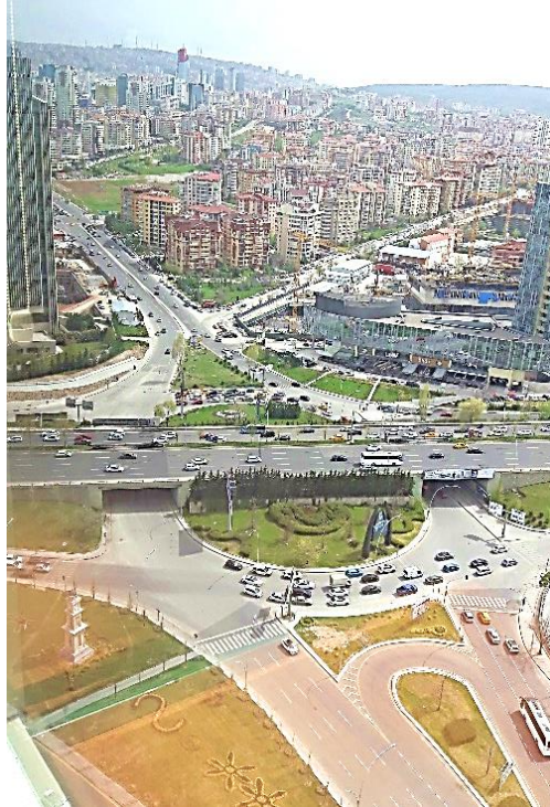
Figure 5.5. Intersection of the main roads
