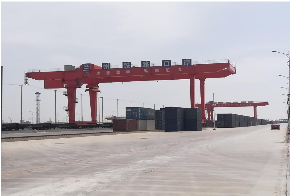
Figure 10 Lanzhou Railway Port, Lanzhou New Area
