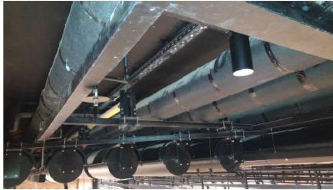
Figure 2.26. Cylindrical variable acoustic elements (Jambrošić, Domitrović & Horvat, 2016)
