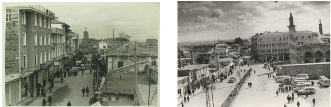
Figure 3.14. Gazi Street Before Widening (left) Gazi Street After Widening (right)
