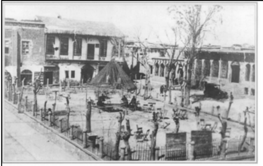
Figure 3.8. Diyarbakir Municipal Park
