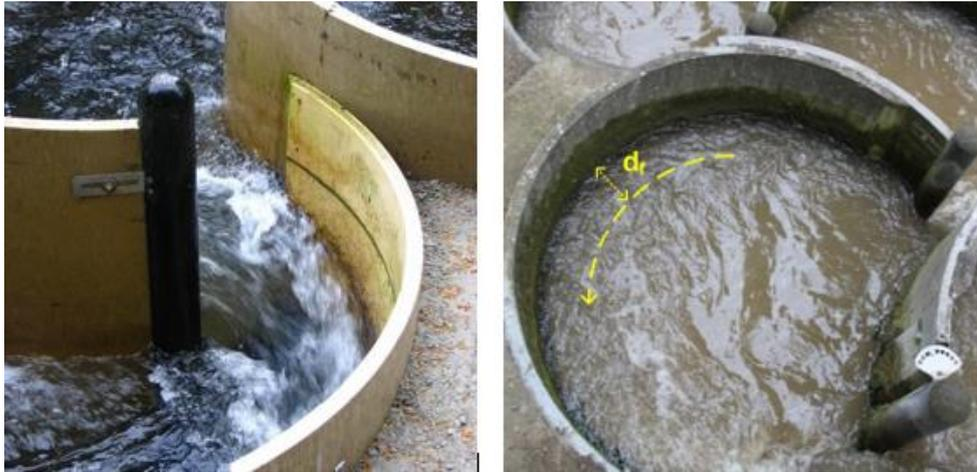
*Figure 1.10.* Current shrinkage around vertical slot (DWA-M 509) (Left); Round vertical slot fish pass on Nethe River,  $d_f$ : distance between theoretical fish migration corridor (yellow arrow) and outer wall of the pool (Right)
