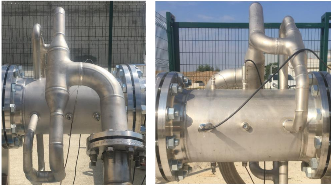
Figure 4-17. Ejector Nozzle Feed Manifold.
