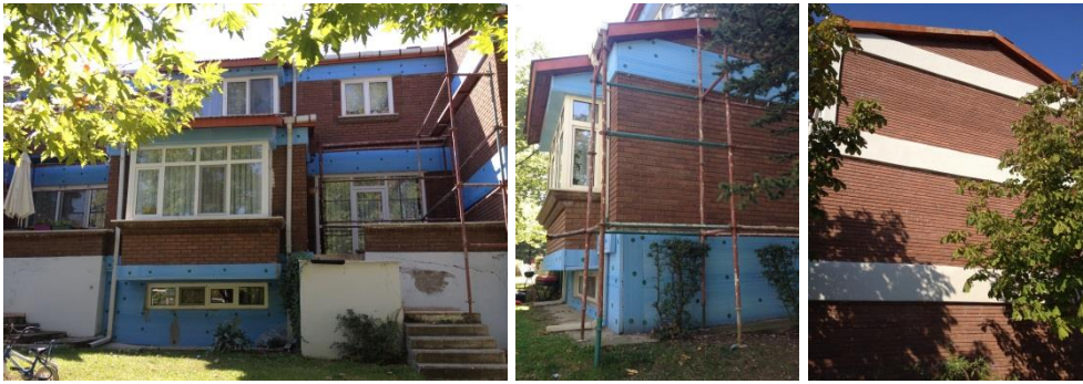
Figure 3.2. Villa type house (B1) during and after externally-insulation of reinforced concrete walls, renovation time: 2014.
