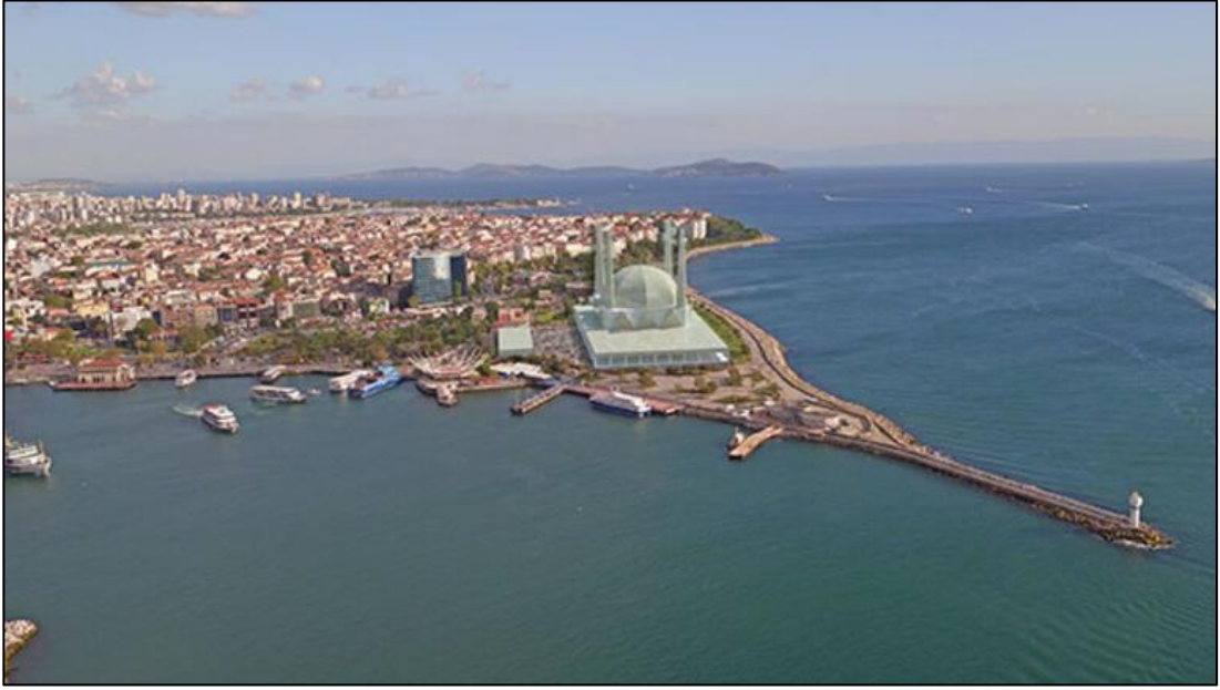
Figure 13: A model of Kadıköy Grand Mosque Project on the coast of Kadıköy, Istanbul (Source: hurriyet.com.tr)
