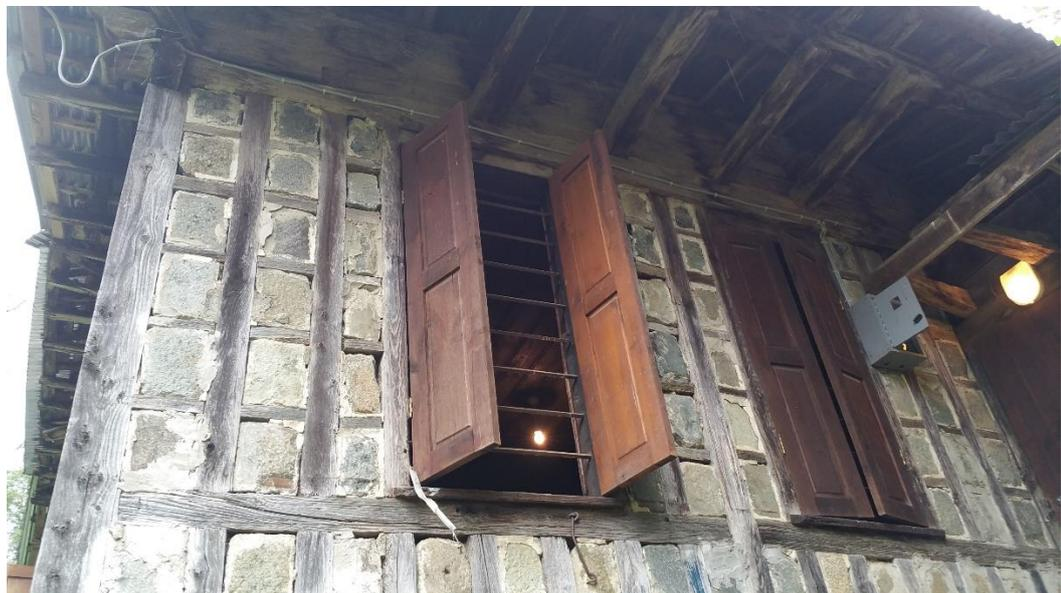
Figure 4.33. Timber shutters and metal guards
