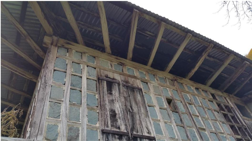
Figure 4.10. Corrugated metal roof covering of Arılı 91
