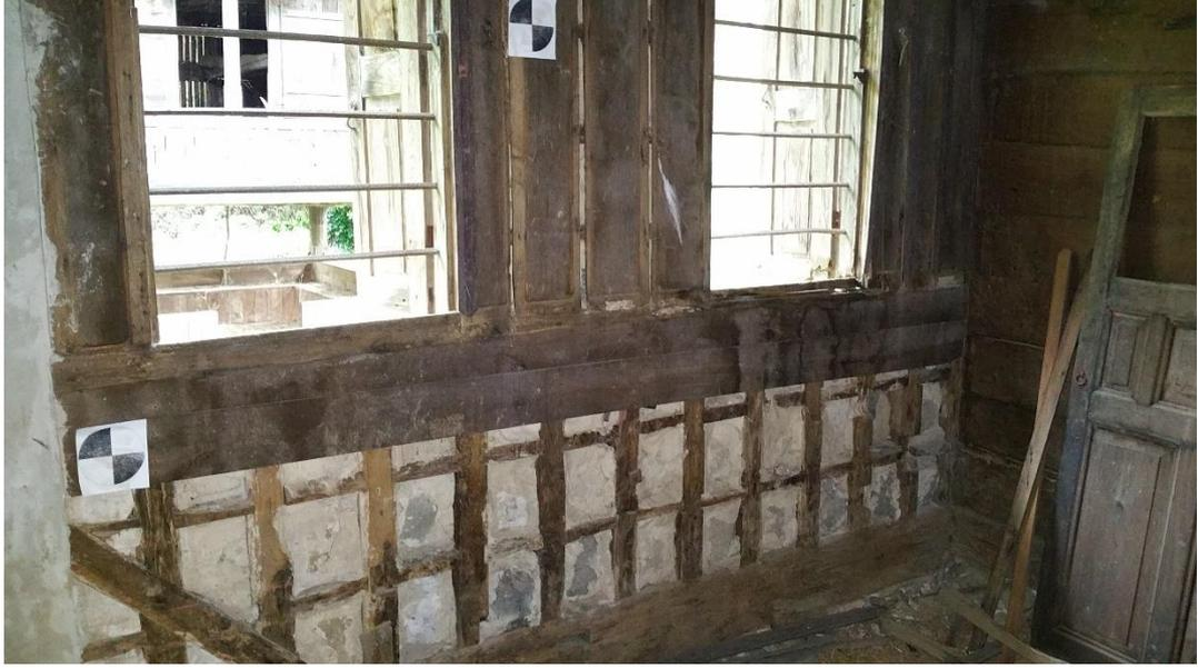
Figure 3.22. Timber plank siding with missing elements in Şenköy 3
