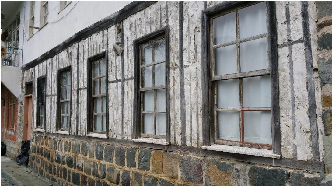
Figure 4.3. Timber frame section of the ground floor walls of Dereüstü 28
