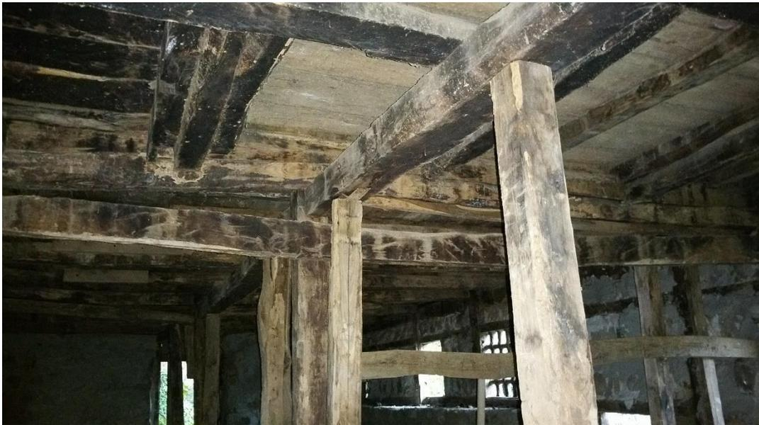
Figure 4.21. Post and beam system in the ground floor supporting first floor
