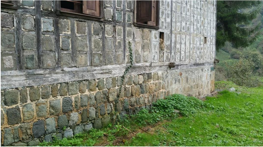
Figure 4.20. Wall plates with kurt boğaz joints
