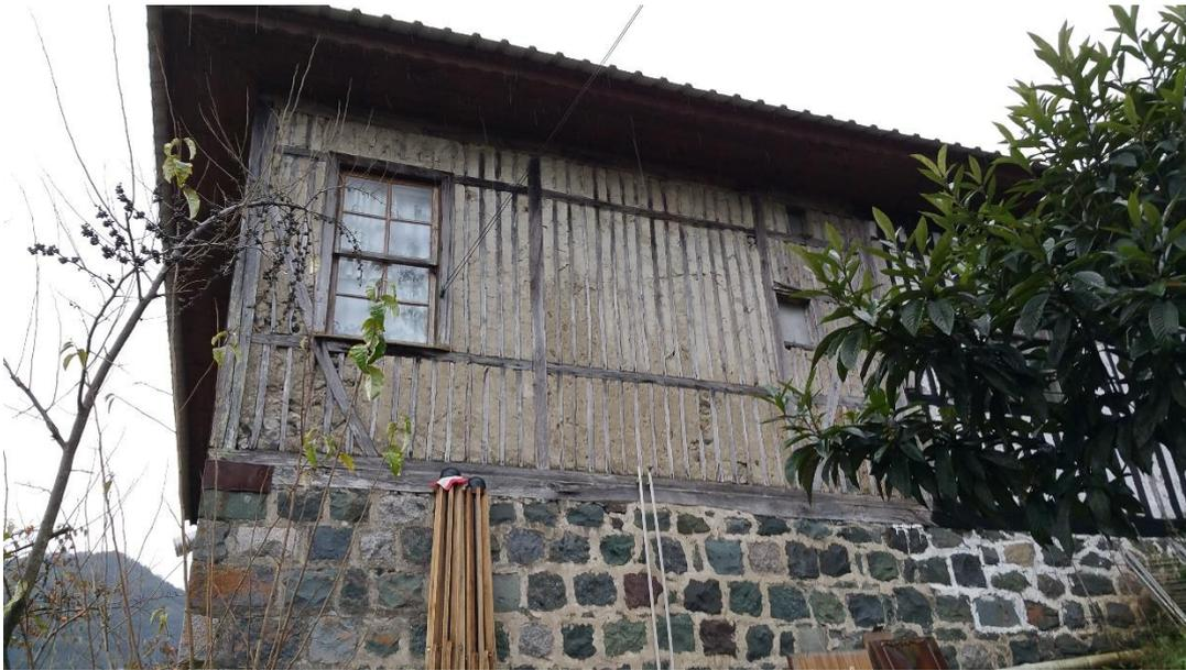
Figure 3.14. Çatma walls of Dereüstü 20
