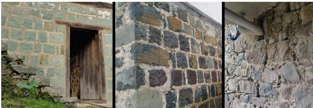
Figure 3.7. Fine cut stone, rough cut stone and rubble stone walls
