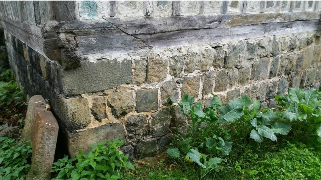
Figure 3.28. Diagonal lengthening details seen on Şenköy 3
