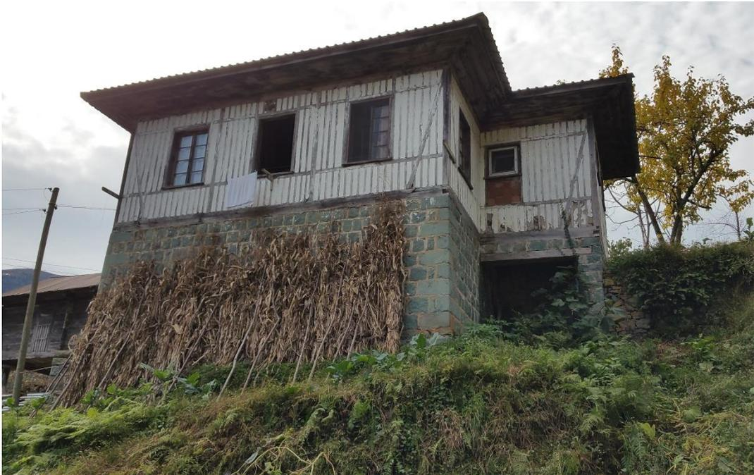
Figure 4.1. Masonry walls of the ground floor and foundation of Arılı 105
