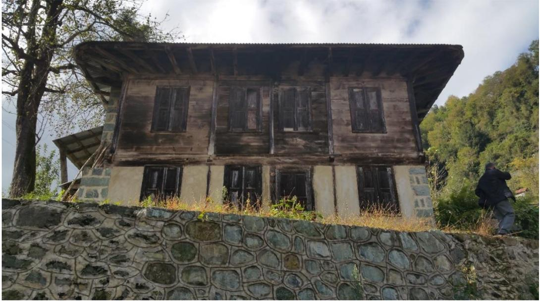
Figure 3.18. Timber infill wall technique in Arlı
