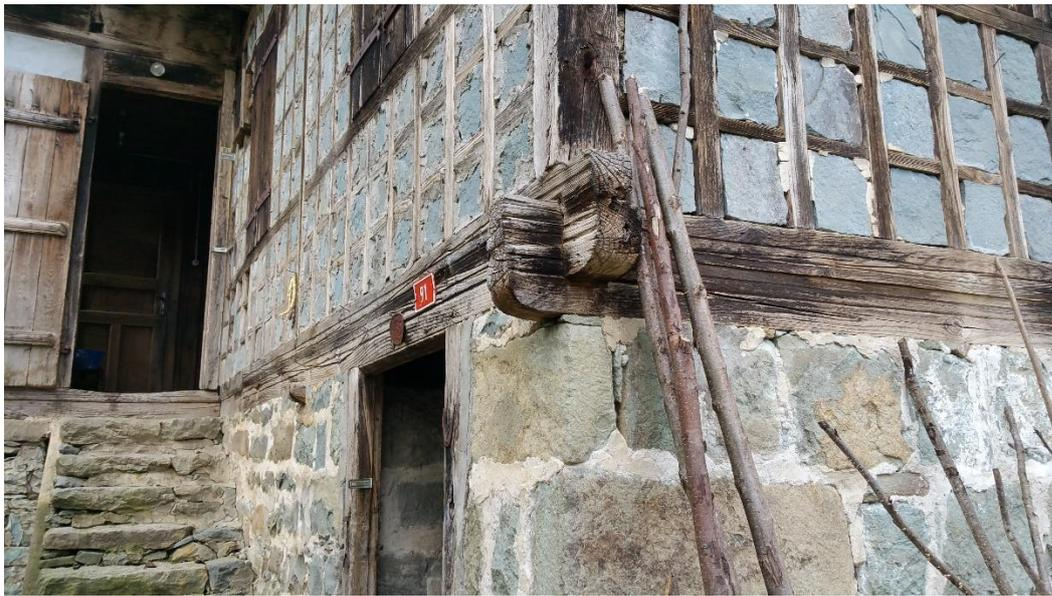
Figure 4.5. Beam joints on Arılı 91
