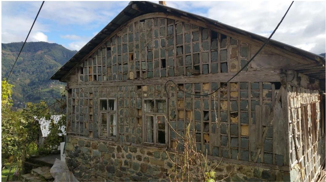
Figure 3.33. A curved sağırcık gable with removed half hip in Arılı
