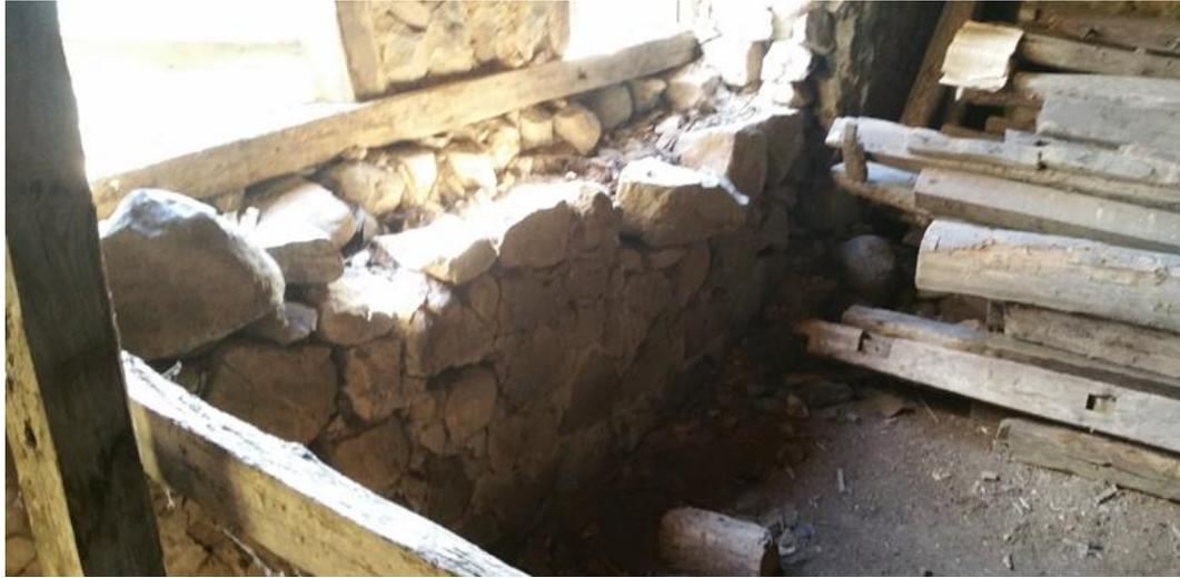
Figure 3.6. Support wall on the ground floor of Şenköy 3
