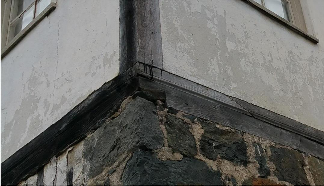
Figure 3.27. Diagonal bonding on Dereüstü 20 with a single timber element that are joined to beams at two sides similarly to the lengthening joint
