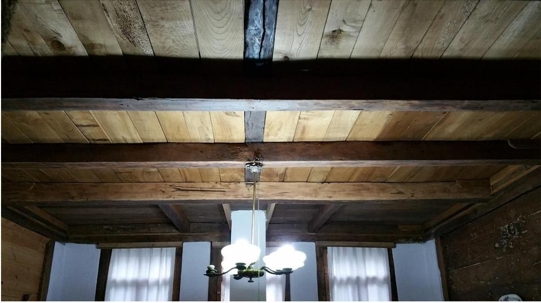
Figure 3.52. Inverted plank ceiling in Dereüstü 20
