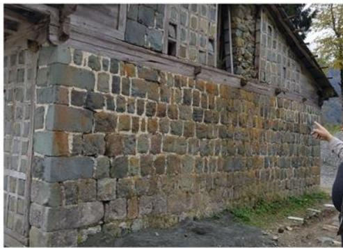
Retaining upper wall up to plate beam - Arılı 47
