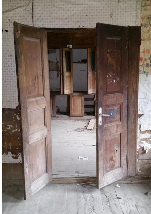
Figure 3.43. Double-wing panel doors in Şenköy 3
