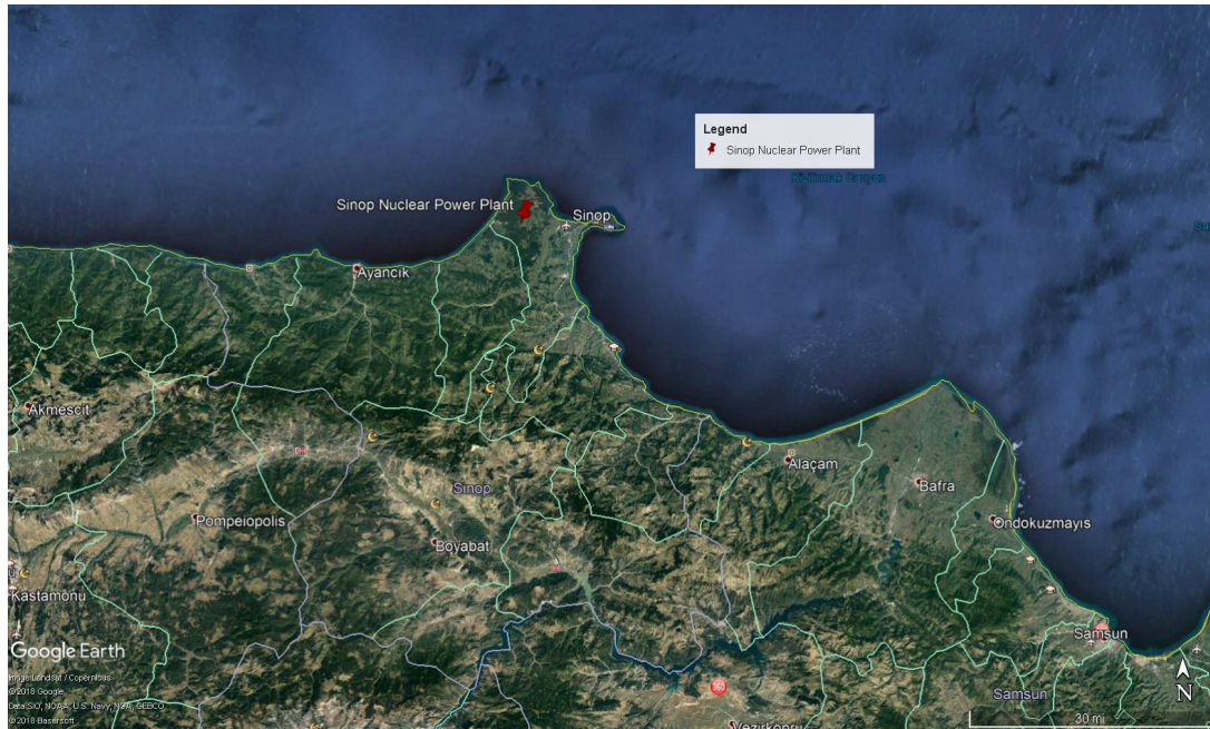
Figure 3.1.2: General view of Sinop-Abalı NPP construction site
