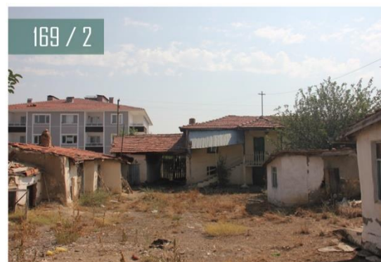
Figure 3-115: Images of mud brick masonry dwellings in the courtyards of stone houses. Source: Author
