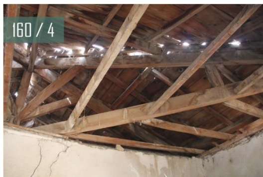
Figure 3-22: Photos showing structural system of the roof and its tile covering.
