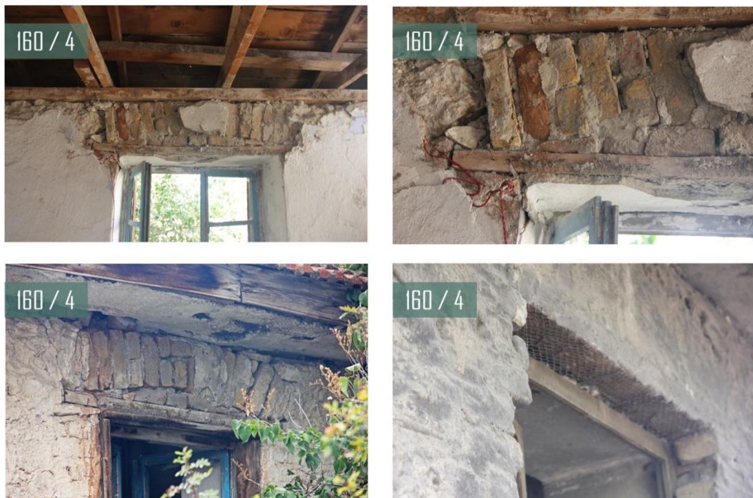
Figure 3-20: Photos showing structural system of window opening.
