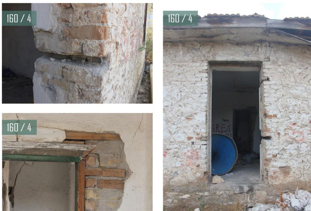
Figure 3-18: Photos showing structural system of door opening. Source: Author
