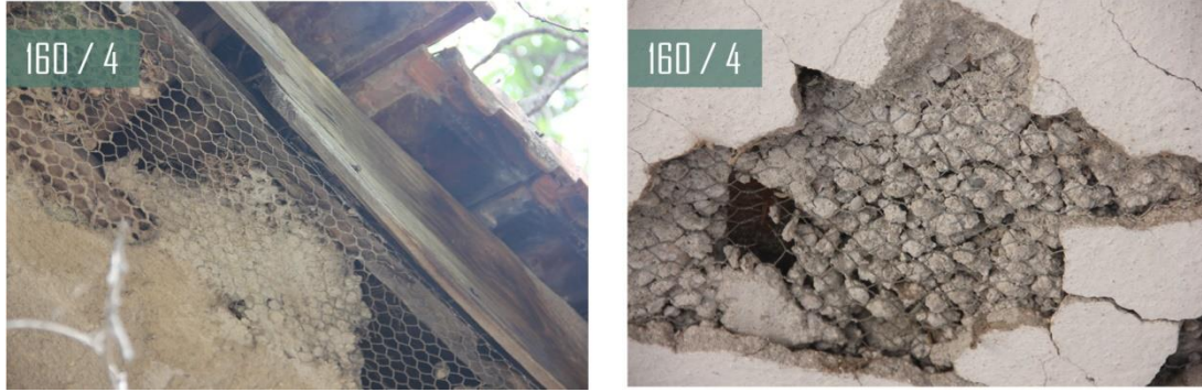
Figure 3-21: Photos showing netting system of the ceiling.
