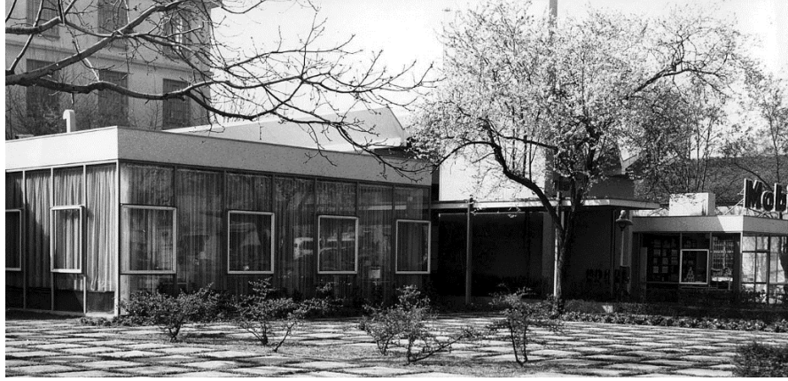
Figure 88 The entrance area of the restaurant next to the oil service station, 1960 Source: Maruf Önal, Courtesy of TMMOB archives
