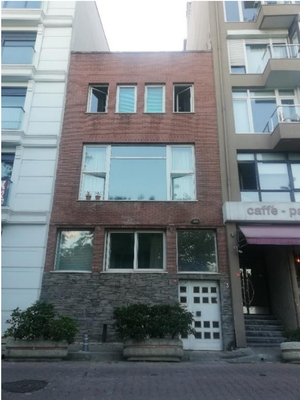
Figure 13 The current outlook of Dr. Belen House after the renovation of the front façade with natural stones, 2019 Source: Author's archives
