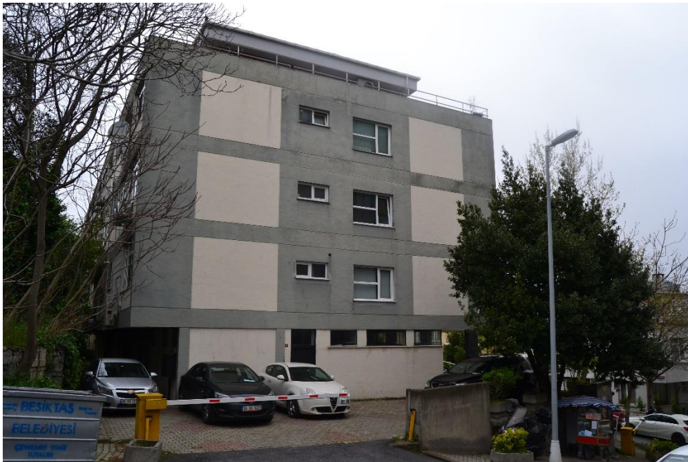
Figure 45 The side façade of Ar Apartment, 2019 Source: Author's archives
