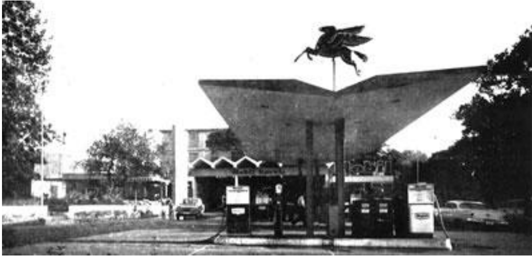
Figure 107 The eave above the service station with Mobil Company's Pegasus logo on the top of the canopy Source: Maruf Önal, 1967
