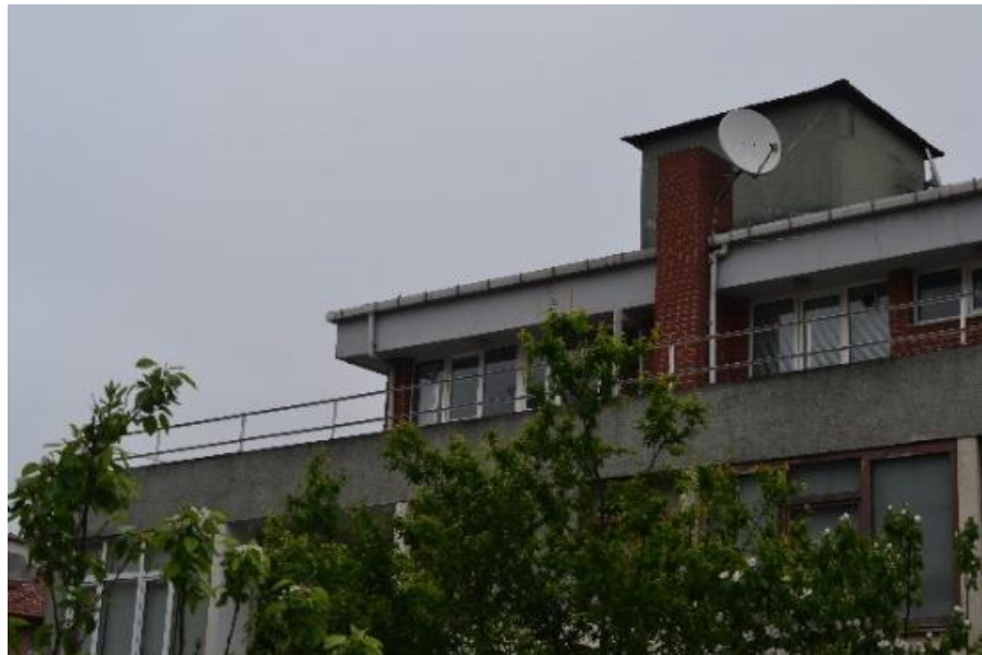
Figure 48 Renovated terrace floor and the back façade of the building, 2019 Source: Author's archives
