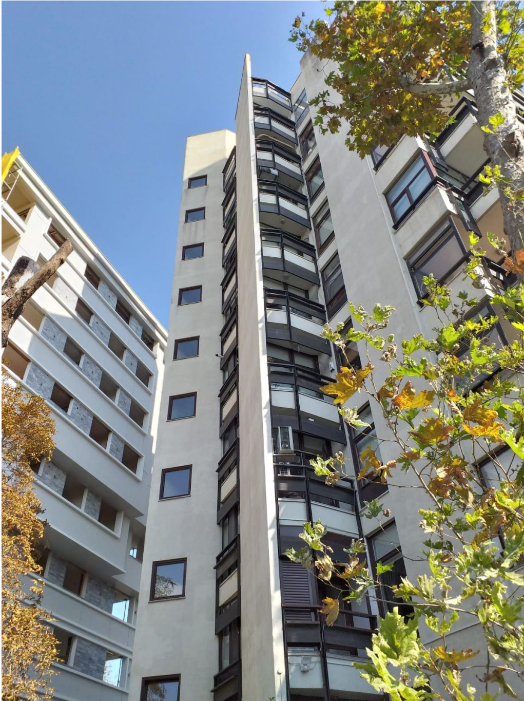
Figure 59 Kaplançalı Apartment, rear facade, 2019 Source: Author's archives
