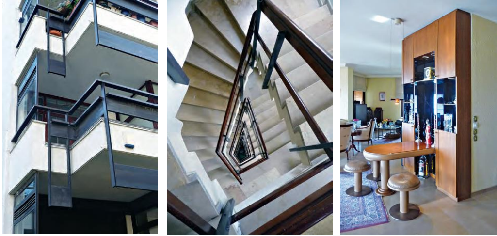
Figure 60 Kaplançalı Apartment, Balcony railing in detail.
