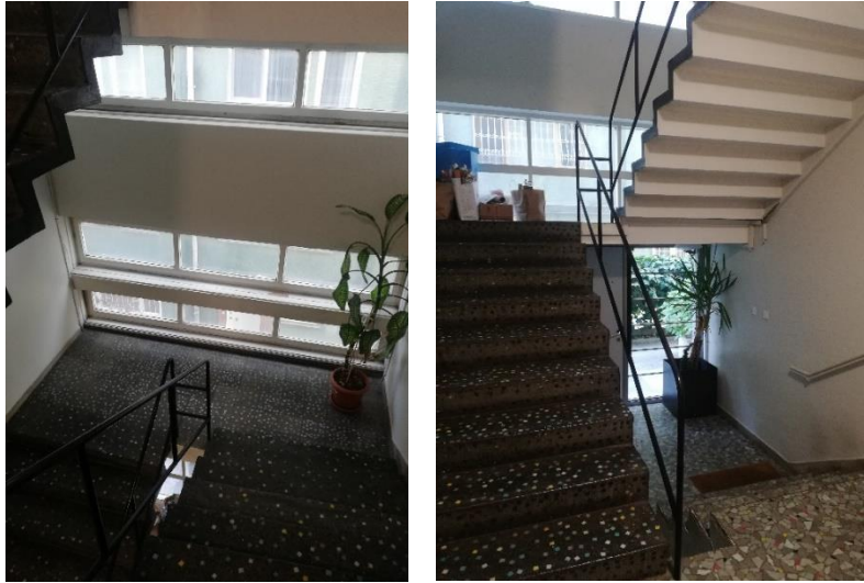
Figure 37 The horizontal windows and staircase inside of the building Source: Author's archives
