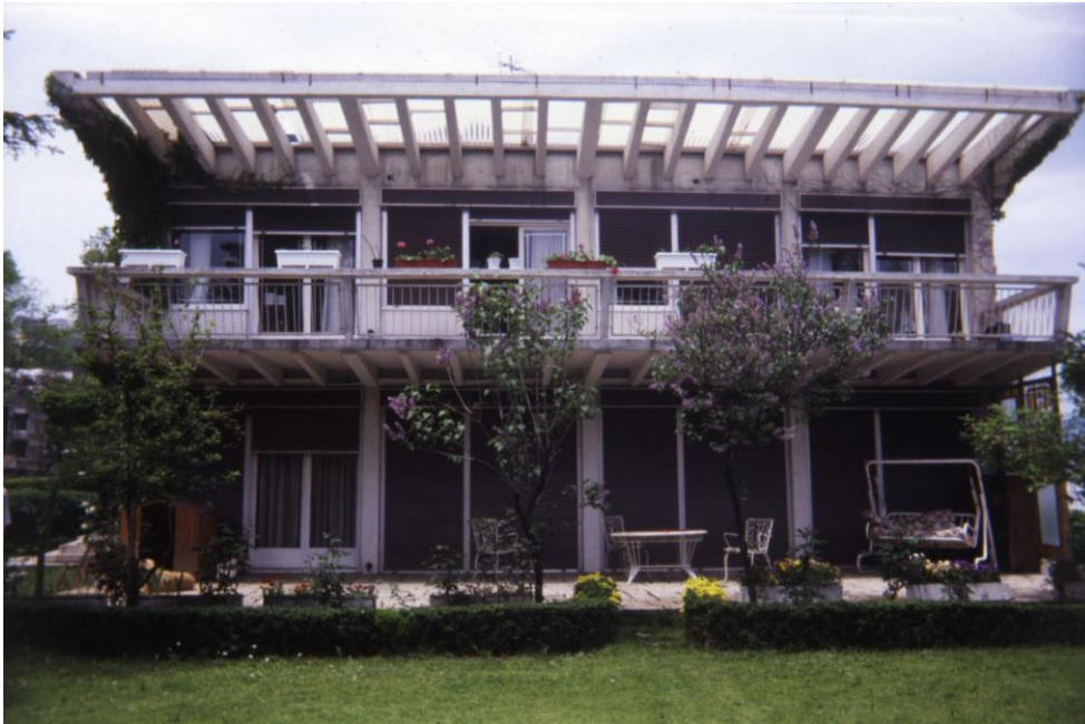
Figure 19 Ardaş Bezaz House, the side front with sun breaker and balconies, 1991 Source: Afife Batur's archives
