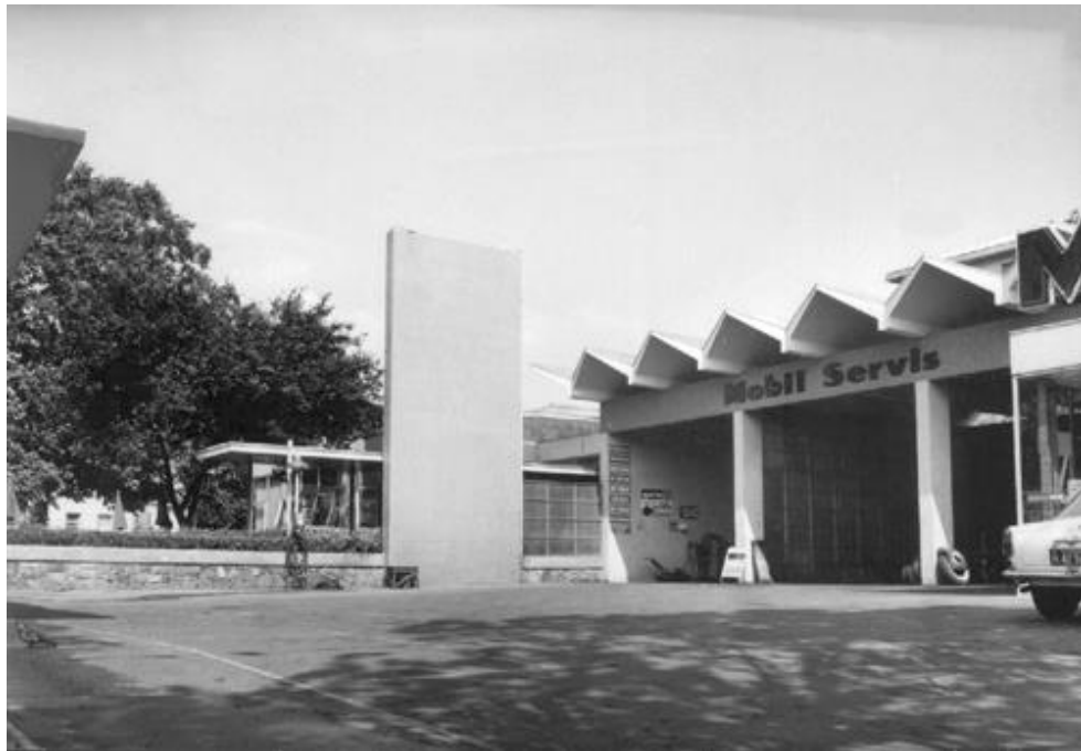
Figure 106 The separator wall between the restaurant area and service station, 1961 Source: Maruf Önal, Courtesy of TMMOB archives
