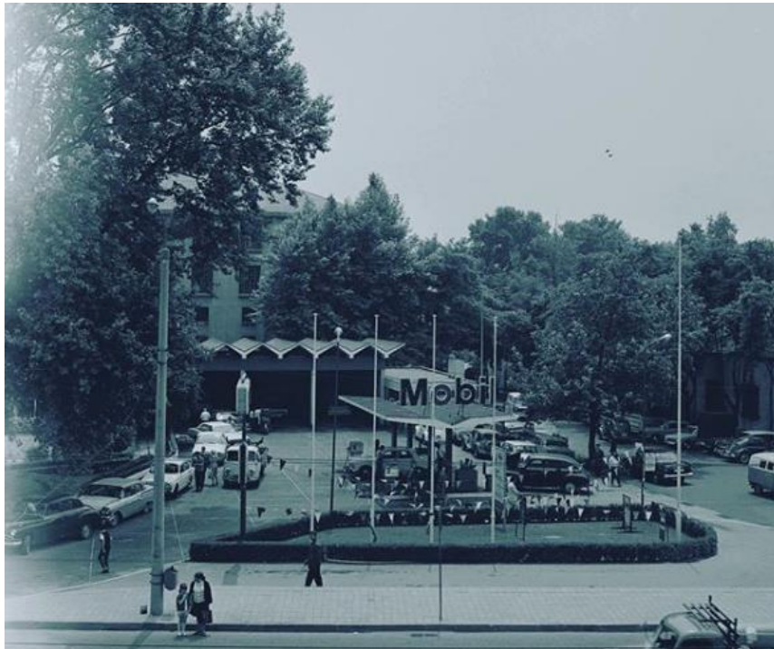
Figure 86 Mobil Service Station area that incorporates Motorest Restaurant, Barbaros Avenue, Beşiktaş, 1960s Source: Anonymous
