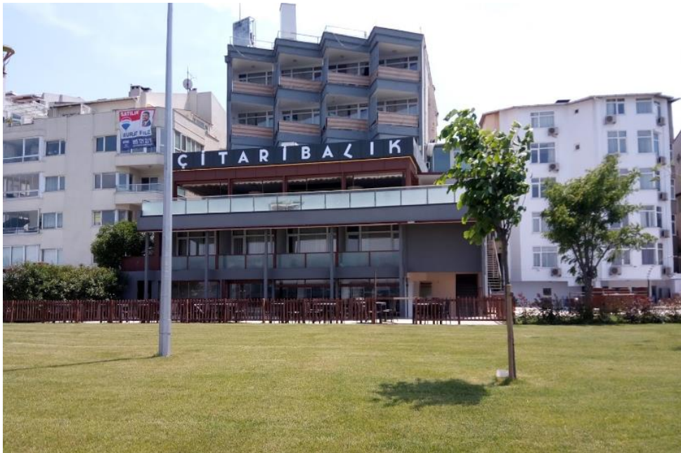
Figure 101 Renovated back facade and the restaurant area of Motel Bekir Source: Sedat Akpınar , 2019. https://goo.gl/maps/nUzSyzVYwgpcSU8
