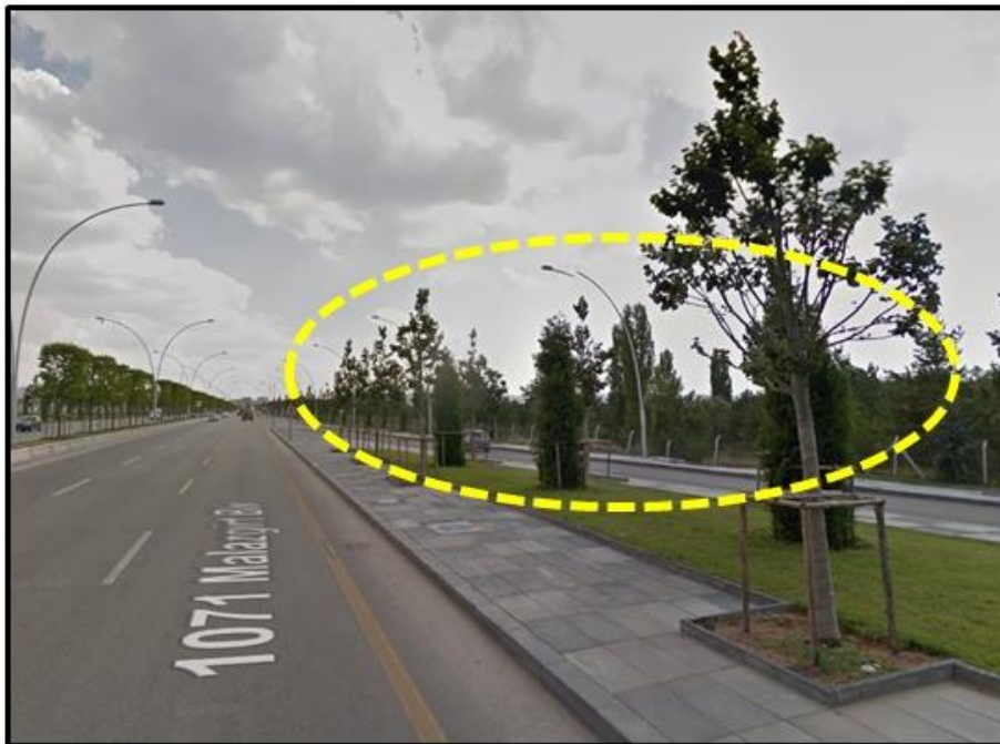
Figure 6.3. Plantings obstructing sight view (Km 0+900)
