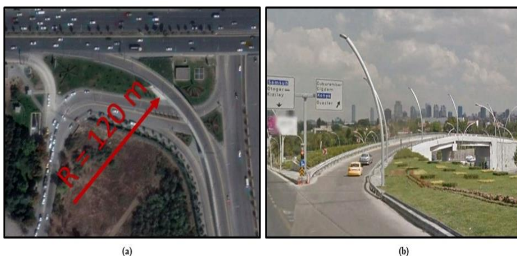
Figure 6.26. Overpassing Bridge Leg on South-west Quadrant of Inonu Boulevard Interchange
