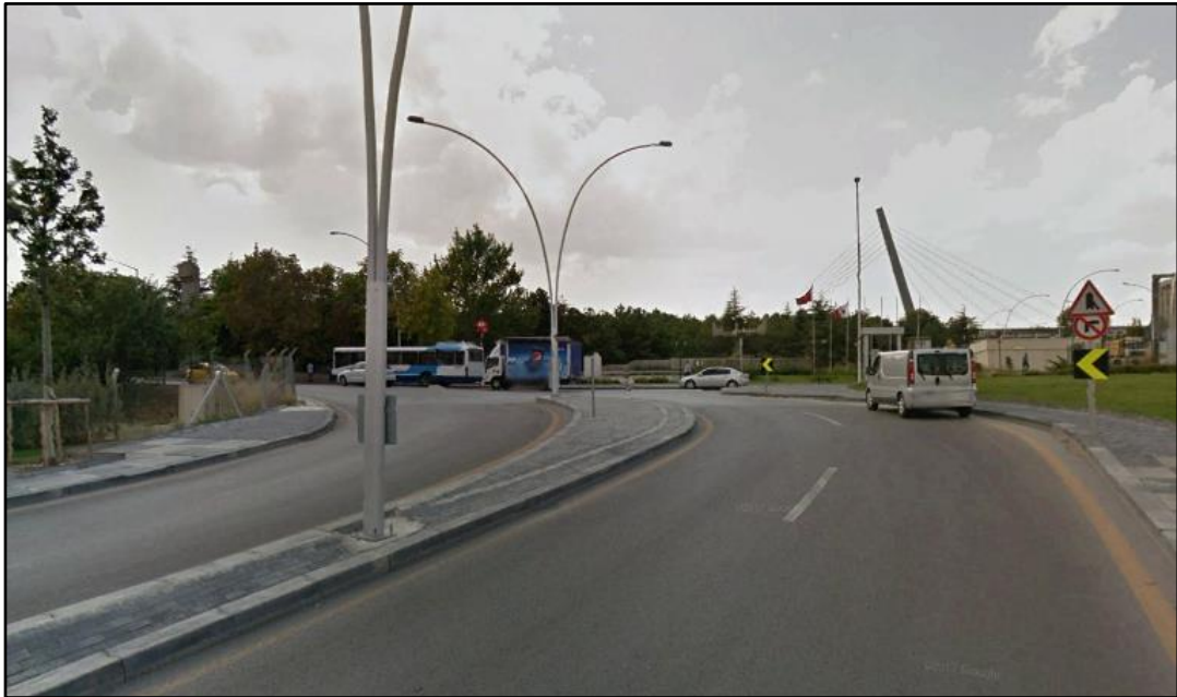
Figure 6.18. Visibility Reduction at A1 Gate Intersection because of Horizontal and Vertical Alignment Layout
