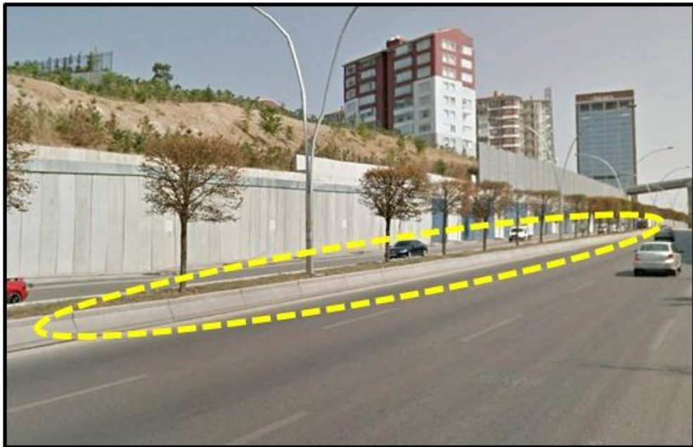
Figure 6.2. Existing Median Barrier (Km 3+300)
