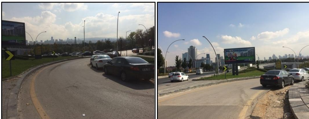
Figure 6.24. Parked Vehicles Obstructing Sight Lines at A1 Gate Intersection
