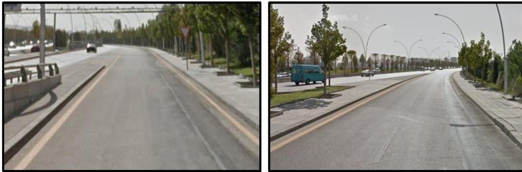
Figure 6.48. Clear Visibility on Acceleration Lanes at Entrance Terminals
