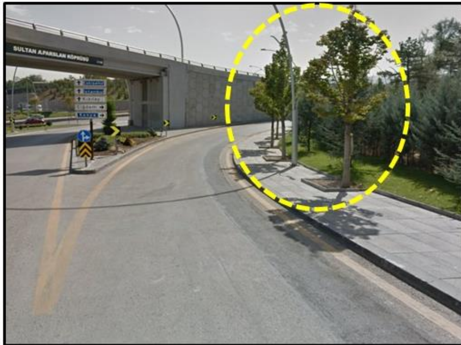
Figure 6.4. Planting that can obstruct sight view in the future after growth (Km 0+350)
