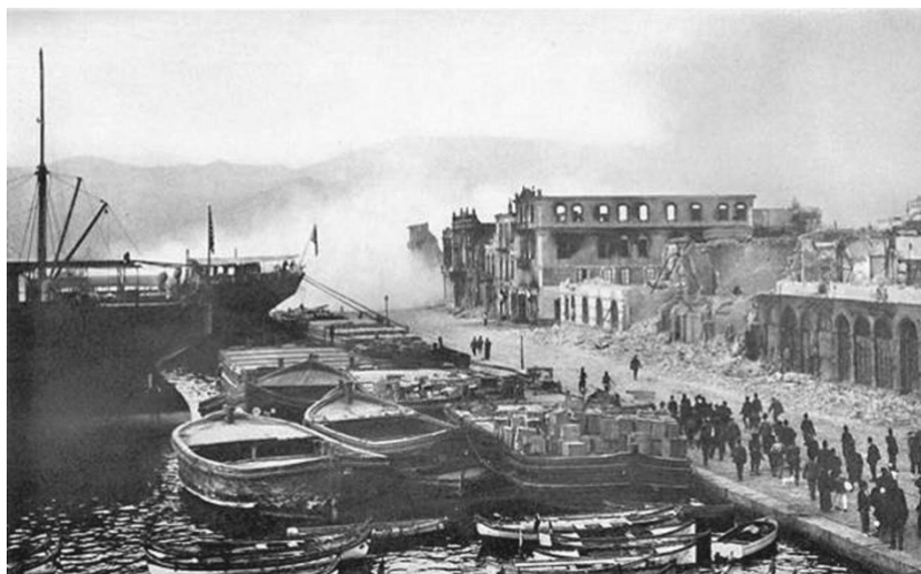
Figure 3.2. Kordon after the fire.
